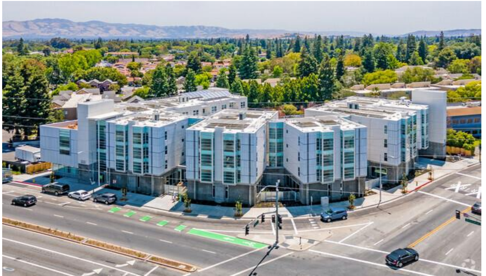
Leigh Avenue Seniors Apartment is a transit-oriented infill project located at 1690 Southwest Expressway, at the intersection of Leigh Avenue and Southeast Expressway. Built by First Community Housing, the project provides 64 units of affordable senior apartments over 6,750 square feet of commercial space. All units are reserved for chronically homeless seniors. (Image Courtesy Apartments.com)
