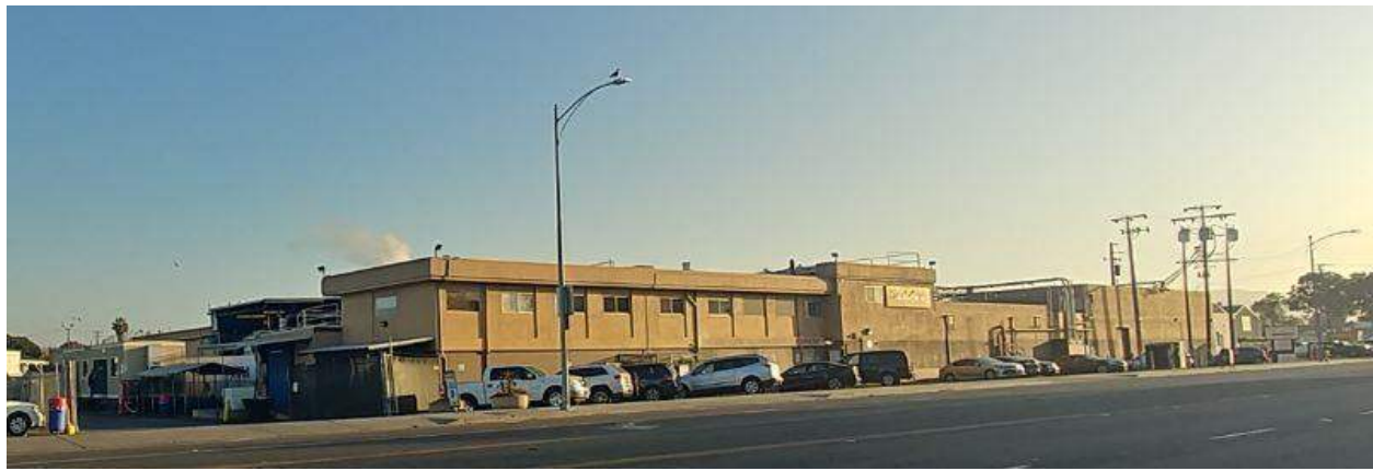
Photograph 1. Front entrance to Site (facing North). 1660 Old Bayshore Highway (1 of 2).
