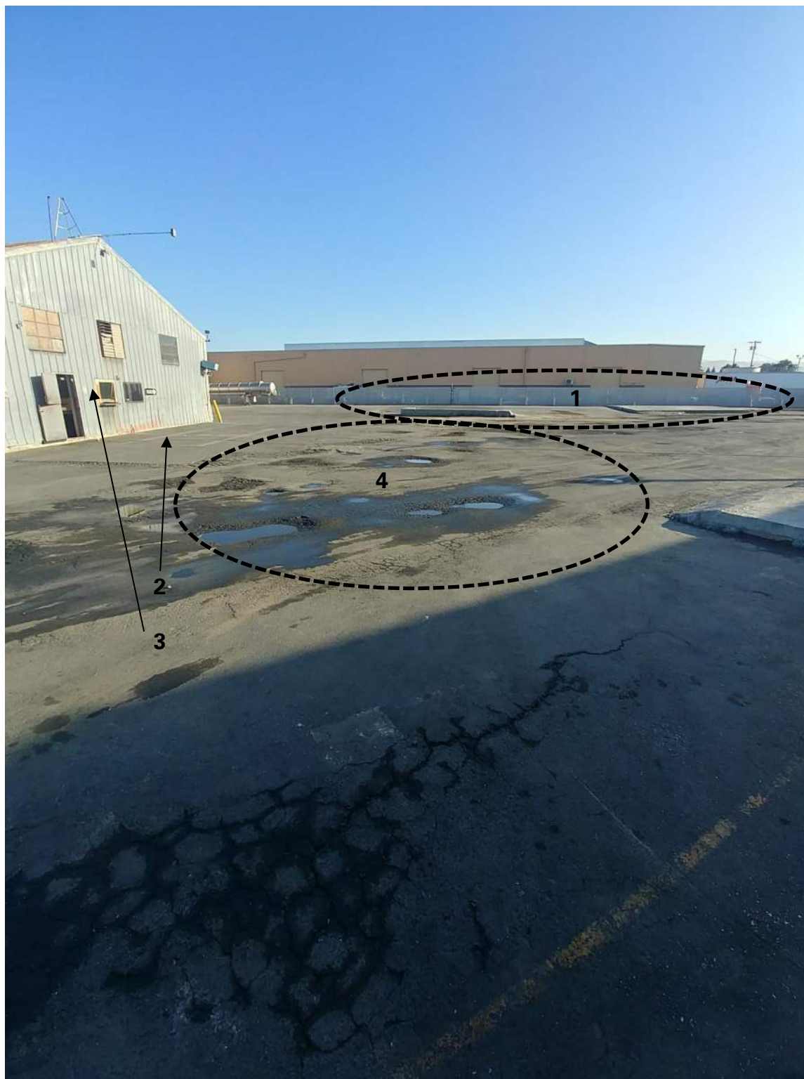
Photograph 20. Feature 1 (circled) is where metal scrap piles have historically been staged. Feature 2 is a truck scale. Feature 3 is a building containing a cashier's office and an employee breakroom. Feature 4 indicates pits in the asphalt containing exposed soil.
