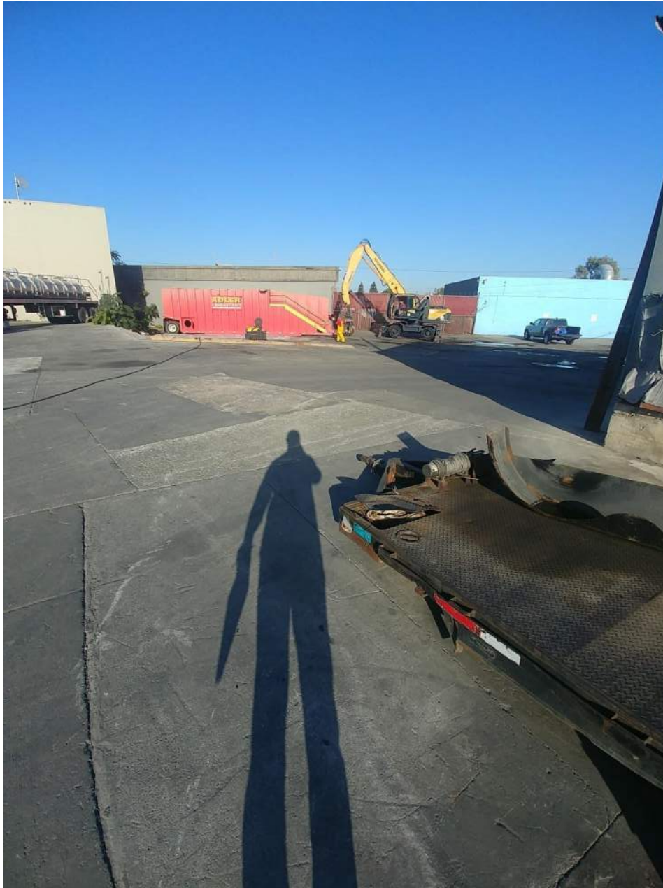
Photograph 19. Recycling Specialists was removing ponded water which had been accumulated into the pictured baker tank on the west side of the site. The water reportedly had ponded around the former metal scrap piles, and contained lubricating oils from the metal cuttings. Refer to features 1 and 4 in Photograph 20.
