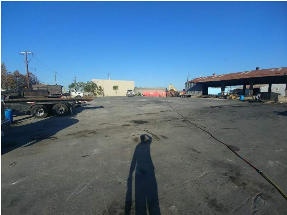
Photograph 18. Facing the western portion of the site, and the footprint of the former Chevron gas station. That area is now covered with a concrete pad approximately six to 12 inches thick.
