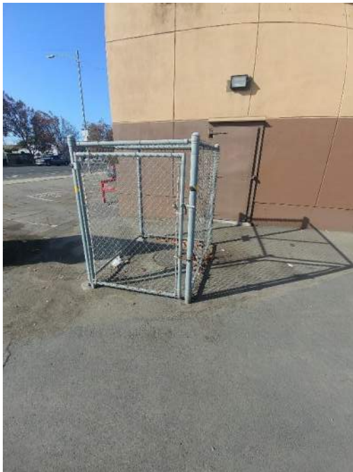
Photograph 4. Manhole access point for sampling stormwater discharge. Facing west, located on the southeast corner of the Smithfield facility.
