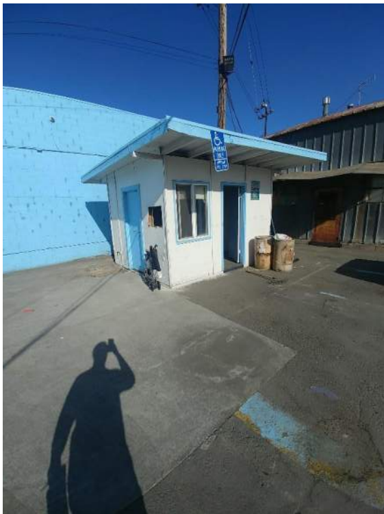
Photograph 28. Guard shack on the west side of the site.
