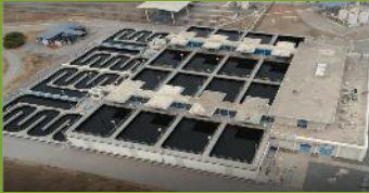
Aerial view of the current filtration area.
