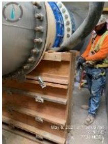
Contractor pouring a concrete pipe support.
