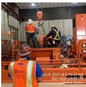
Contractors disassembling a blower in the Tertiary Blower Building.
