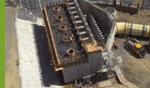
Progress on the raw sewage pump station
