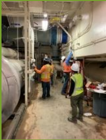
Contractors pressure testing air supply lines.
