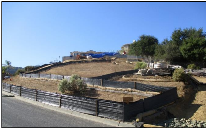
Effective BMPs installed on hill at construction site.
