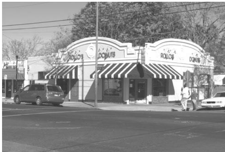
Rollo's Donuts at North Thirteenth and Jackson Streets – as upgraded under the City's façade improvement program
