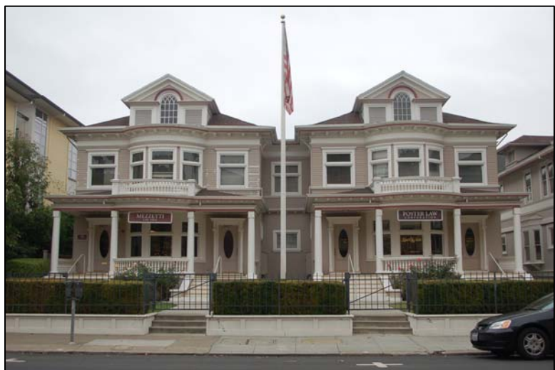
Figure 15: 31 East Julian Street
