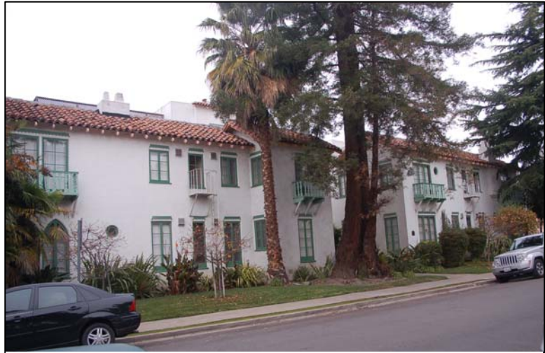
Figure 16B: Barcelona Apartments, 15 Hawthorne Way
