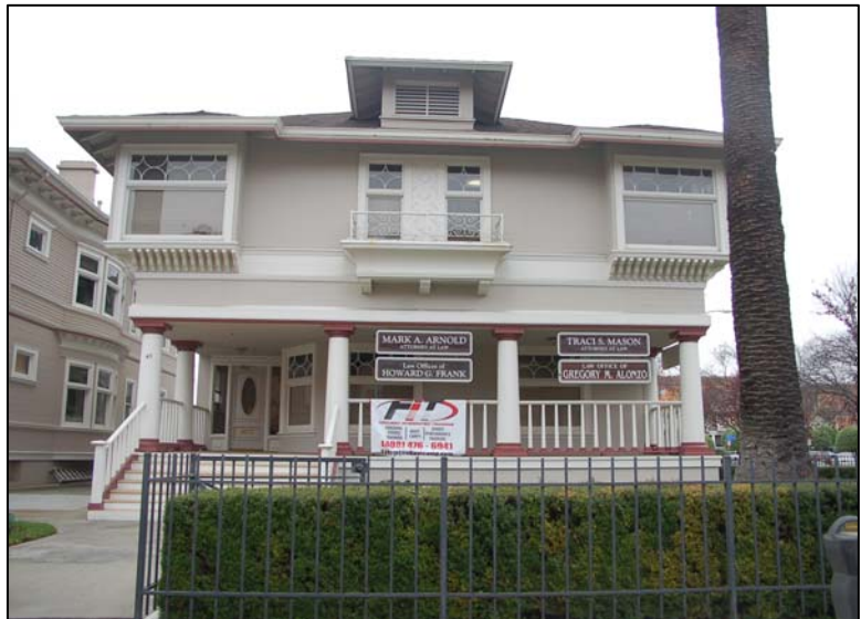
Figure 11: 45 East Julian Street
