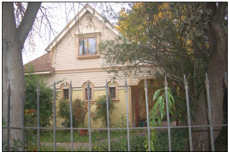
Figure 12: The Leib Carriage House, 60 North Keeble Avenue, ca. 1898
