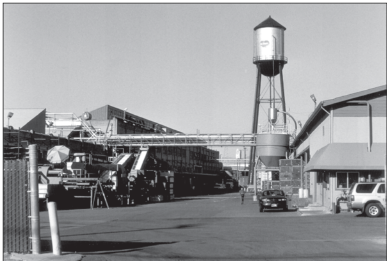
Figure 16: Calpak Plant No. 3, 801 Auzerais Avenue, main cannery complex with water tower and office building (right)
