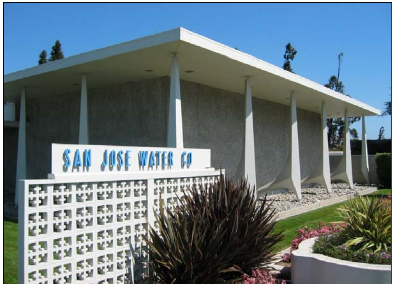
Figure 25: San Jose Water Company Bascom Avenue Pumping Station, 1999 West San Carlos Street, ca. 1960 (Photo courtesy of Heather David)
