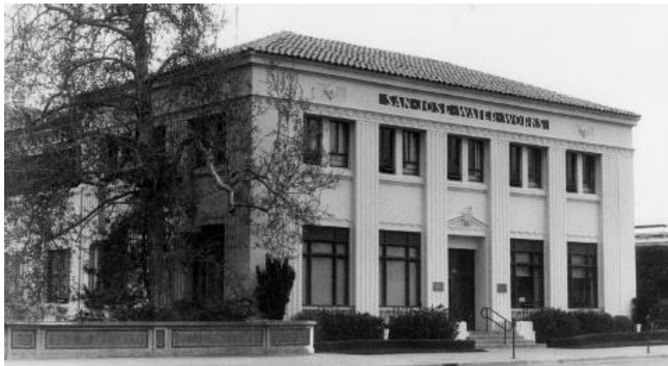
Figure 22. San José Water Works, 1934 ( History San José, American Institute of Architects - Santa Clara Valley Collection, 2008-131-48 ).
