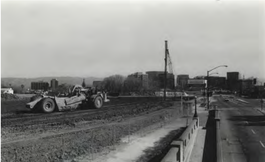
Figure 28. San Jose Arena under construction, 1991 (History San José, Leonard McKay Collection, 2004-17-1103).
