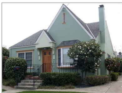
554 Hull Ave. George L. Keesling House
