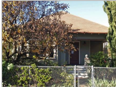
897 Delmas Ave. SP Railroad Agent's House
