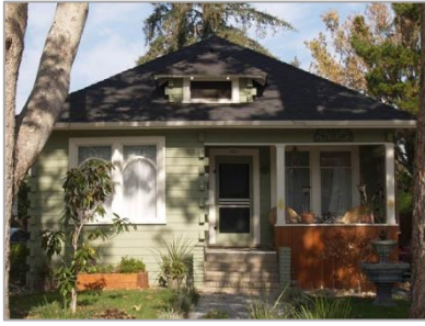
423 Marshall Ave. Petersen House
