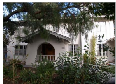
1050 Bird Ave. James Chilton House
