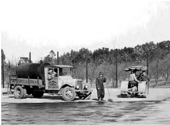
Figure 12 Road construction in Santa Clara County.
