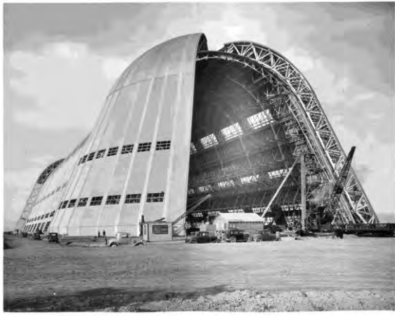
Figure 13 Moffett Field's Hanger One under construction, ca. 1933.
