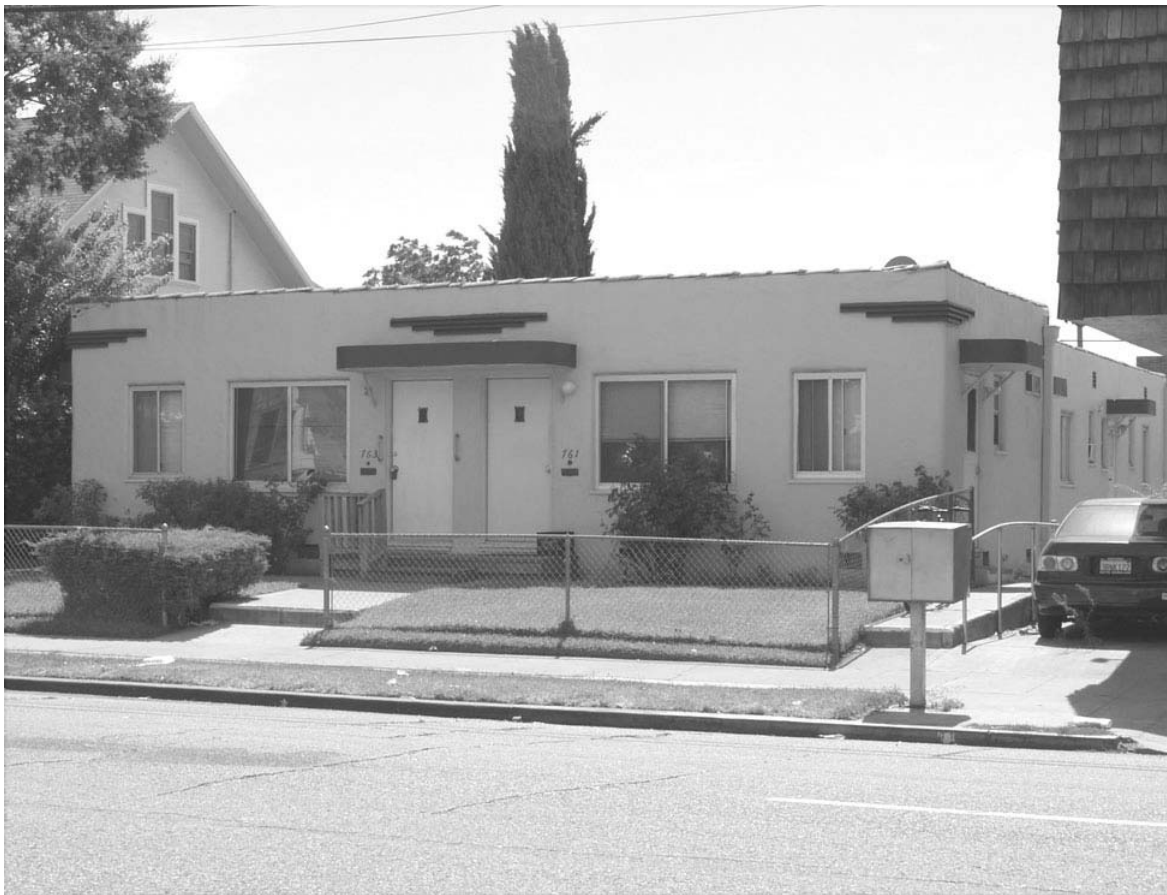
5-plex at 767-771 South Second St. Original windows have been replaced with vinyl inserts.
