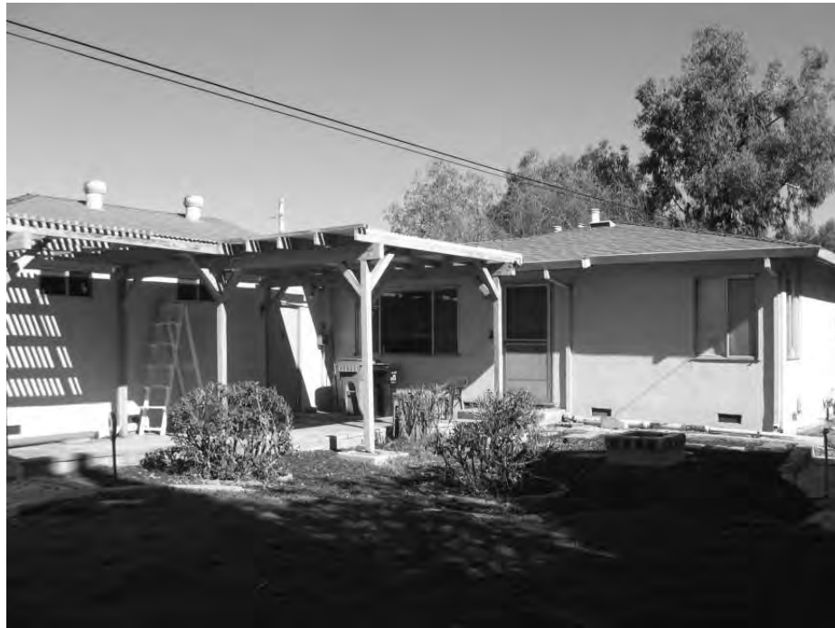
Photo 3: View of the front entry and arbor addition.
