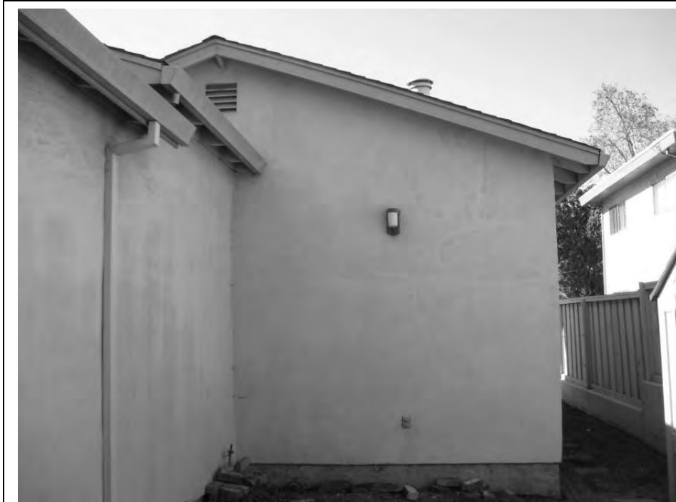
Photo 11: View of rear of the garage addition.
