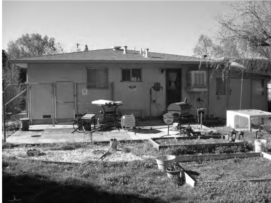
Photo 7: View of the rear facade of the residence.
