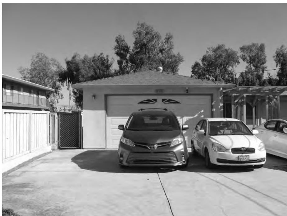
Photo 2: View of the garage addition (1995).
