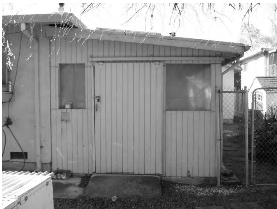
Photo 8: View of informal shed-roof addition on the rear facade.
