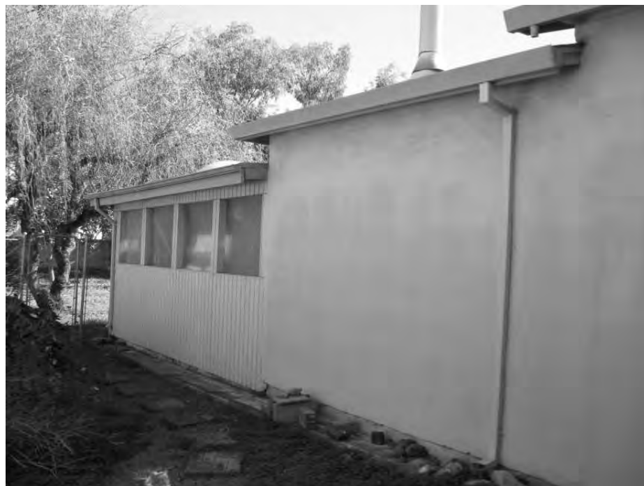
Photo 10: View of roofline suggesting multiple rear additions.
