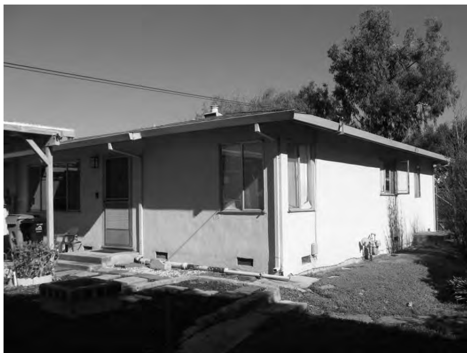
Photo 4: Oblique view of the original portion of the home.
