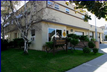
Major Repairs at Fire Stations 3, 10, and 30
