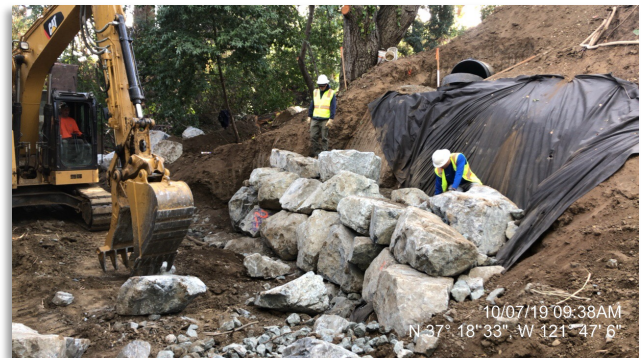
An outfall being rehabilitated on Thompson Creek
