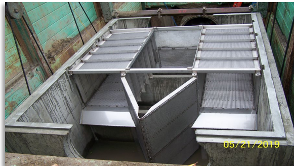
LTC device installation near Coyote Creek
