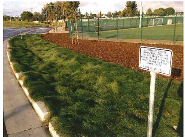
CIP 4949 - Watson Remediation and Ph. I Improvements
