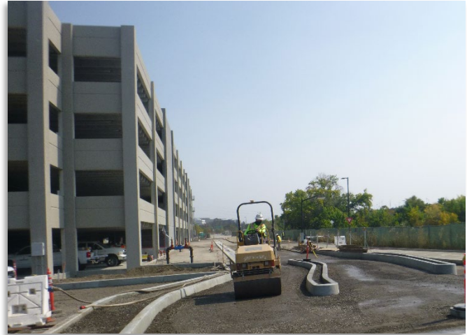
Economy Lot 1 Parking Garage under construction
