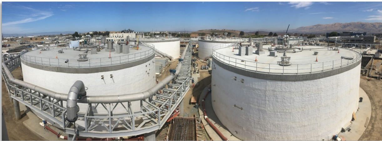
Upgraded Digester Facilities
