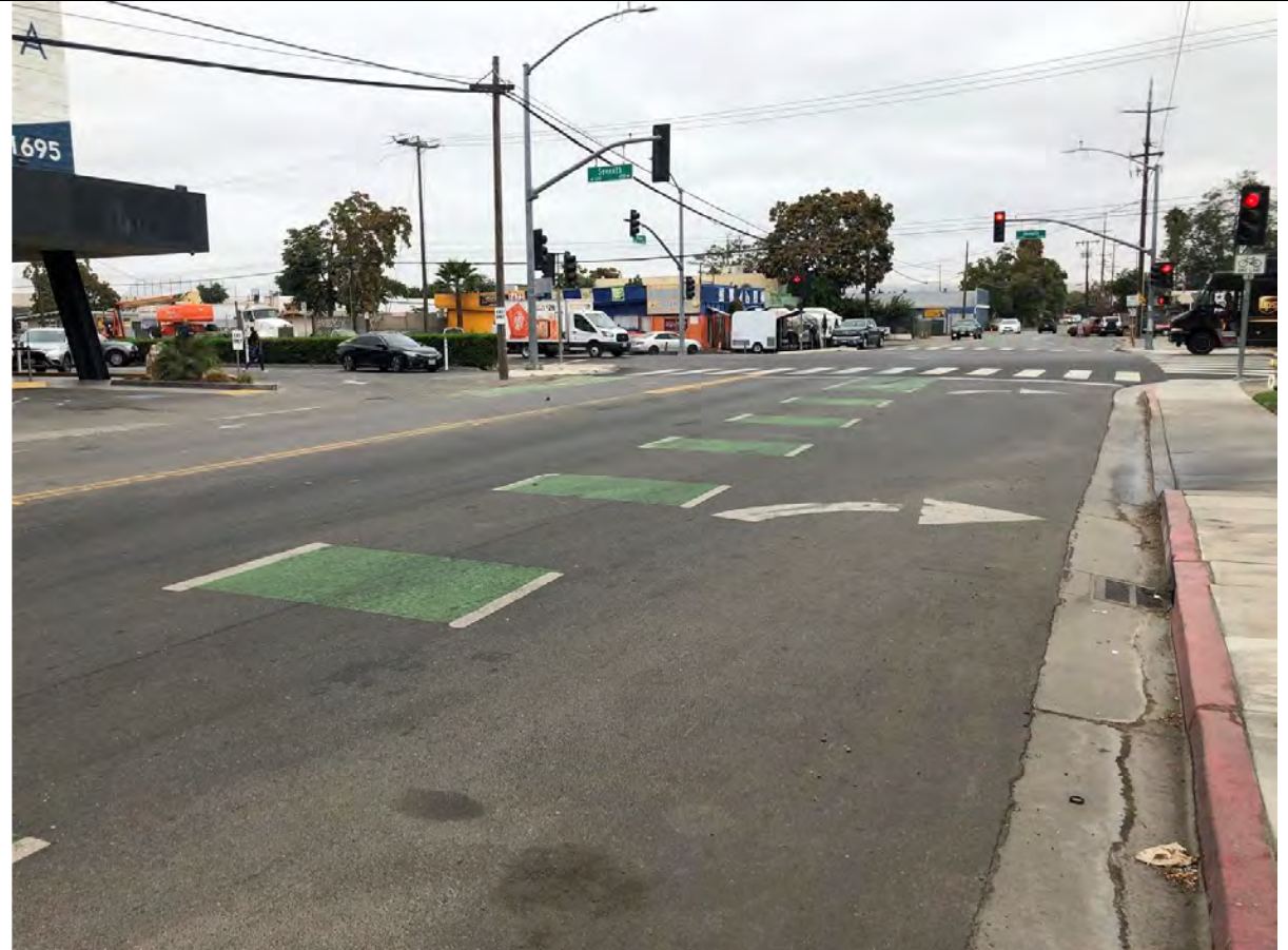
Phelan Ave, facing NE toward intersection with S. 7 th St. Note: No sidewalk on NW side of Phelan, bike lanes on Phelan Ave end to NE of intersection.
