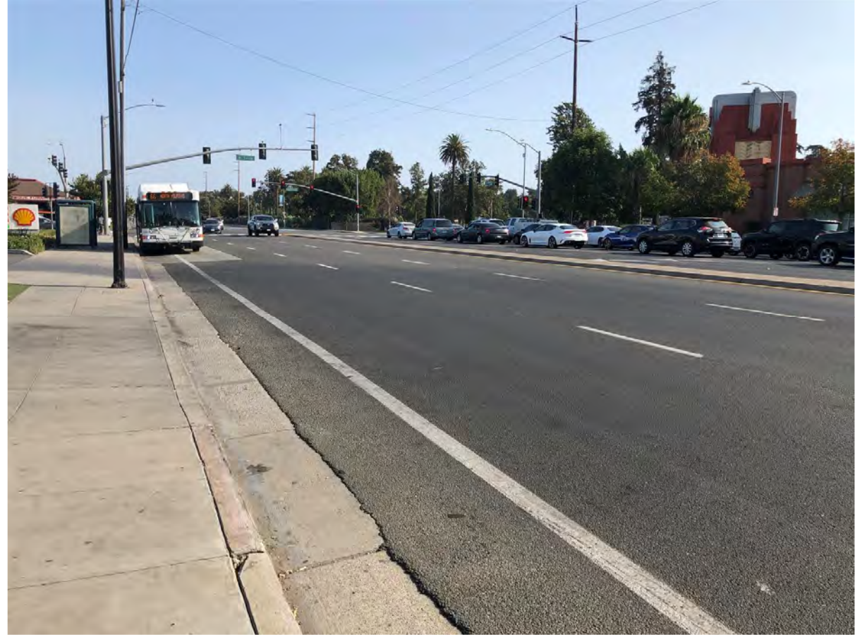
Monterey Rd, facing SE towards intersection with Tully Rd. Note: no dedicated turnout for bus stop.
