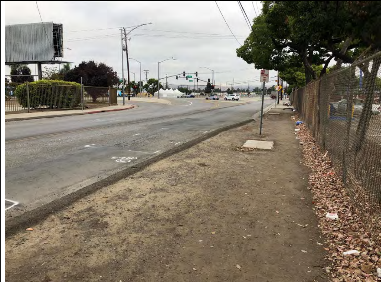
Old Tully Rd, facing N toward intersection with Tully Rd. Note: tight right turn from E-bound Tully Rd onto SW-bound Old Tully Rd creates poor visibility for merging. Also note intermittent sidewalks on Old Tully Rd.
