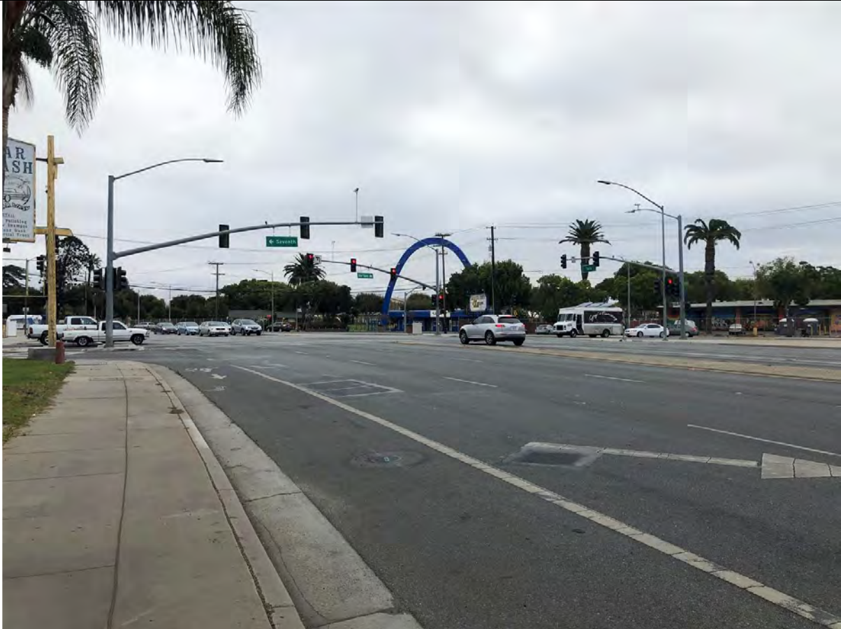
Tully Rd, facing E toward intersection with S. 7 th St. Note loss of right-hand lane on W-bound Tully Rd (right/foreground).
