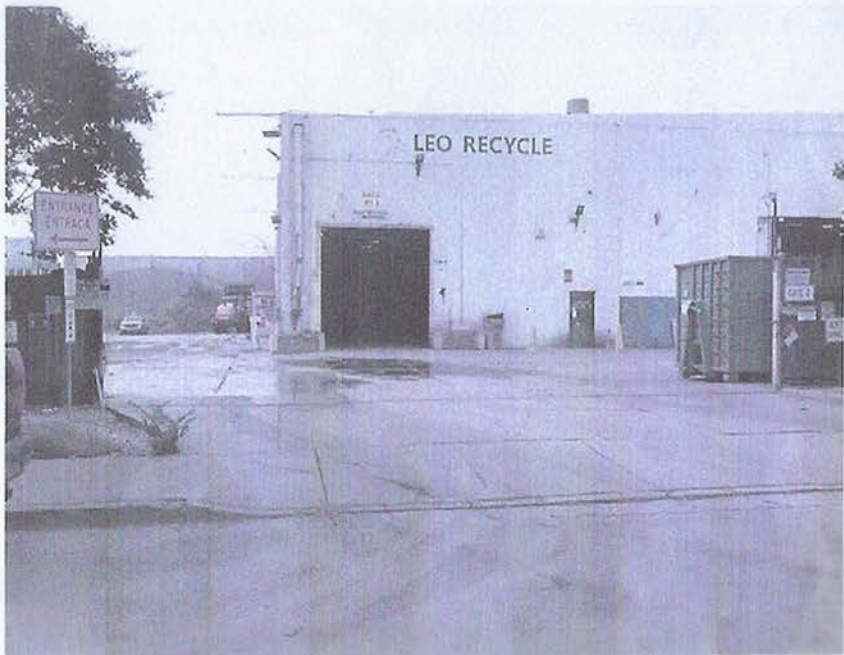
GATE #2 Looking At Entrance To AREA #1
