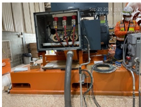
Contractor at the Tertiary Building Blower #5
