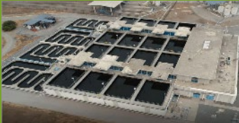
Aerial view of the current filtration area.
