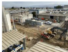
Contractors completing grading and draining near Digester 5.
