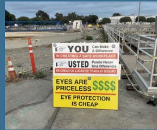
Safety signage at Nitrification Clarifier Rehabilitation Project
