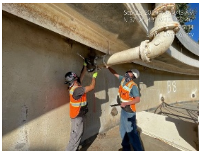
Contractor reconnecting scum piping in a clarifier.
