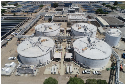
Aerial view of the Digester and Thickener Facilities Upgrade Project.
