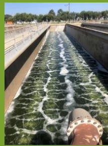
Testing diffuser replacements in the Nitrification Tanks.
