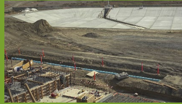
Contractors re-constructing the berm for the Emergency Overflow Basin
