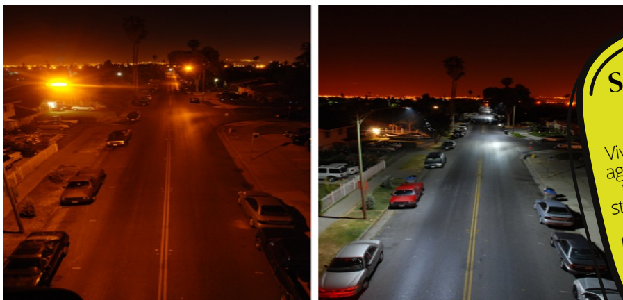
Here is a before and after picture of a street with upgrades LED fixtures
