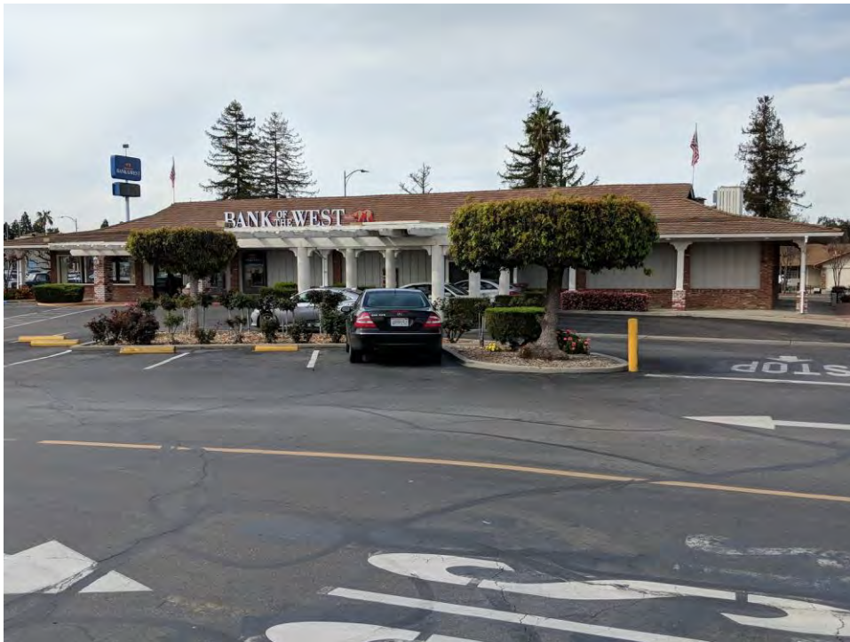
West Detached Building (Bank) with Modern Arbor. Viewed facing North. July 2018.
