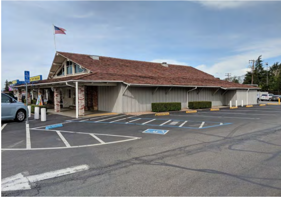
Side of the Southern-most Retail Space. Viewed facing Northeast. July 2018.
