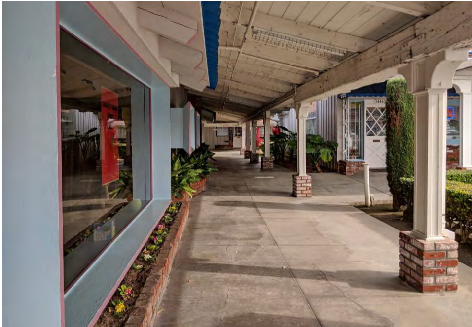
Interior Courtyard of Southern Wing. Viewed facing Southeast. July 2018.
