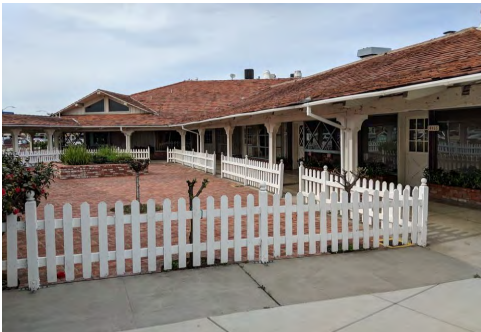
South Courtyard of Central Wing. Viewed facing North. July 2018.
