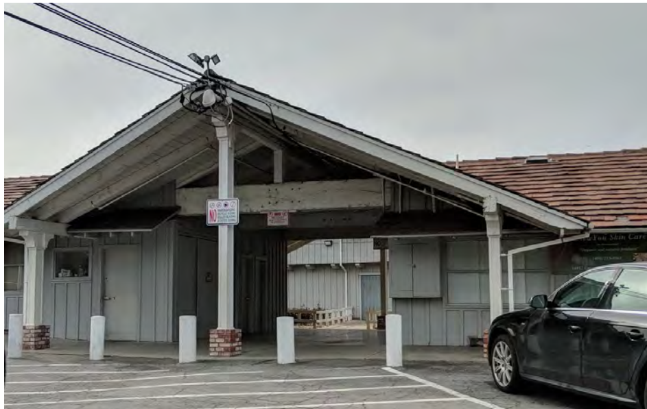
Outside (Rear) View of Gabled Portico into Southern Courtyard. Viewed facing Northwest. July 2018.
