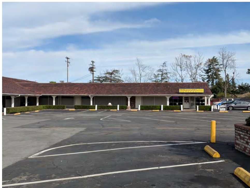
Northeast Detached Retail Building, South Wing. Viewed facing East. July 2018
