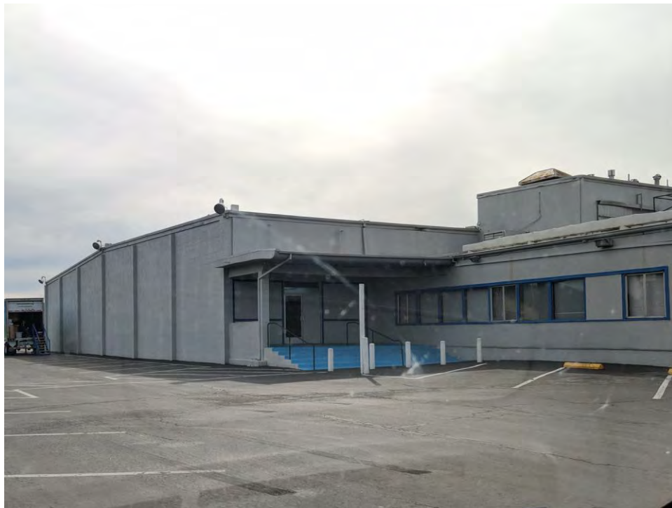
Side of Bowling Alley Wing. Viewed facing Southwest. July 2018.
