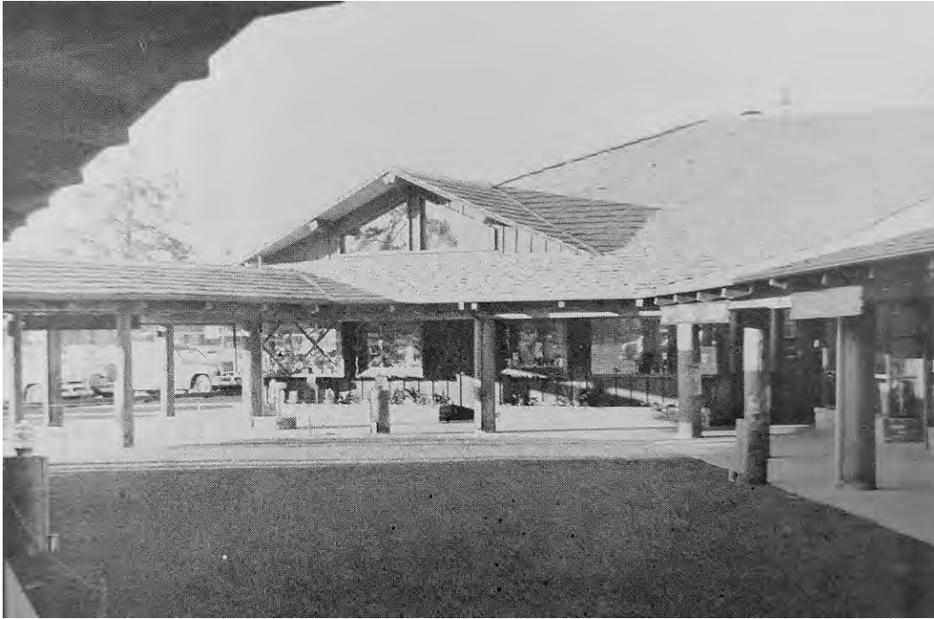
Interior court area
