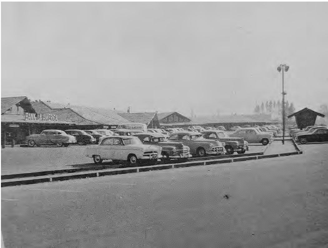
View facing southeast from near carousel sign
