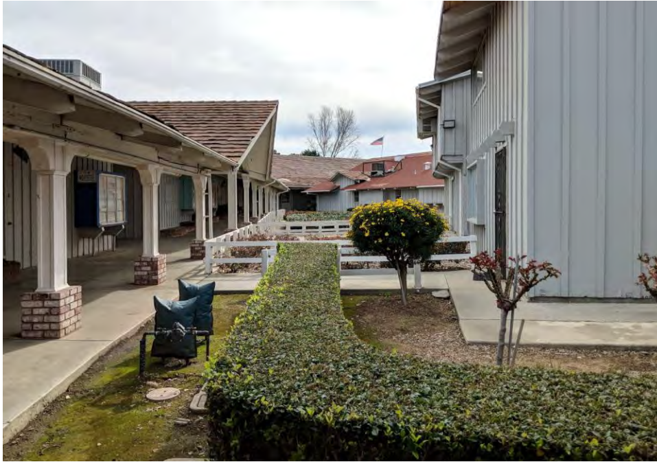
Interior Courtyard of Southern Shops Featuring Gabled Breezeway Portico. facing Southwest. July 2018
