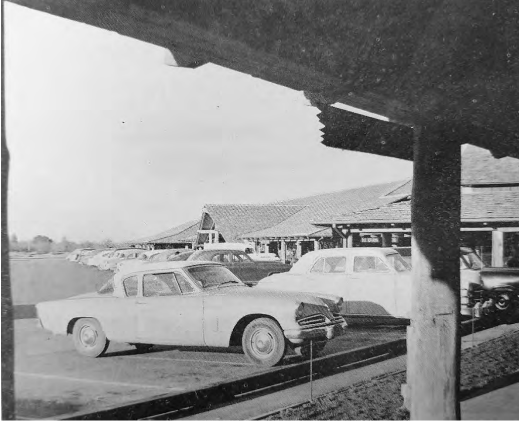
View from south wing facing north.
