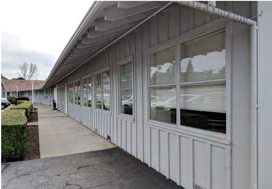
Rear of Southern Shops. Viewed facing Southwest. July 2018
