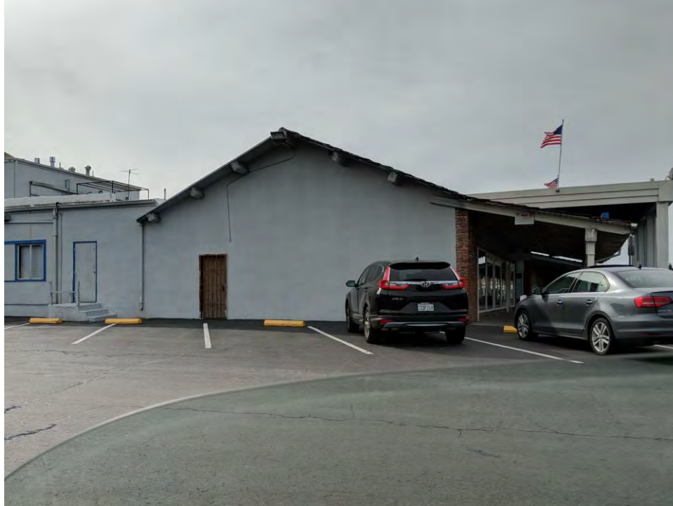
East Side of Bowling Alley Wing. Viewed facing west. July 2018.
