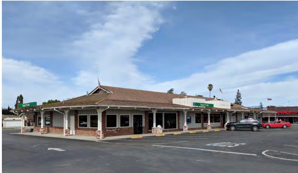
Retail Building to East of Driveway Entrance. Viewed facing Northeast. July 2018.
