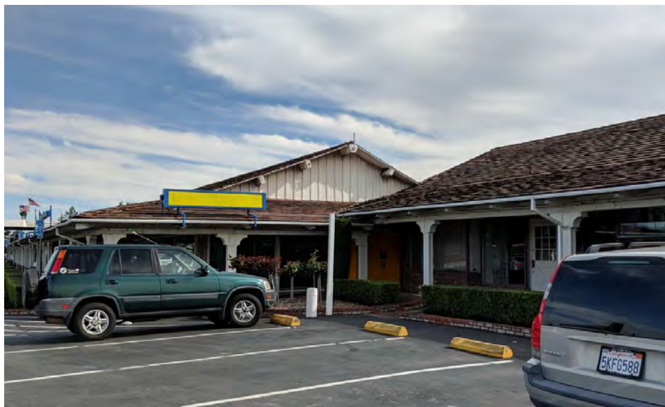
Jog in Building Alignment Along North Corridor. Viewed facing East. July 2018.
