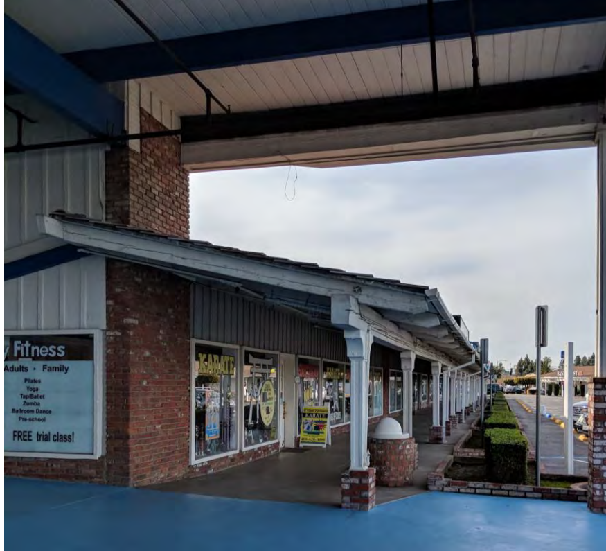
North Main Circulation Collonade From Bowling Portico. Viewed facing West. July 2018.
