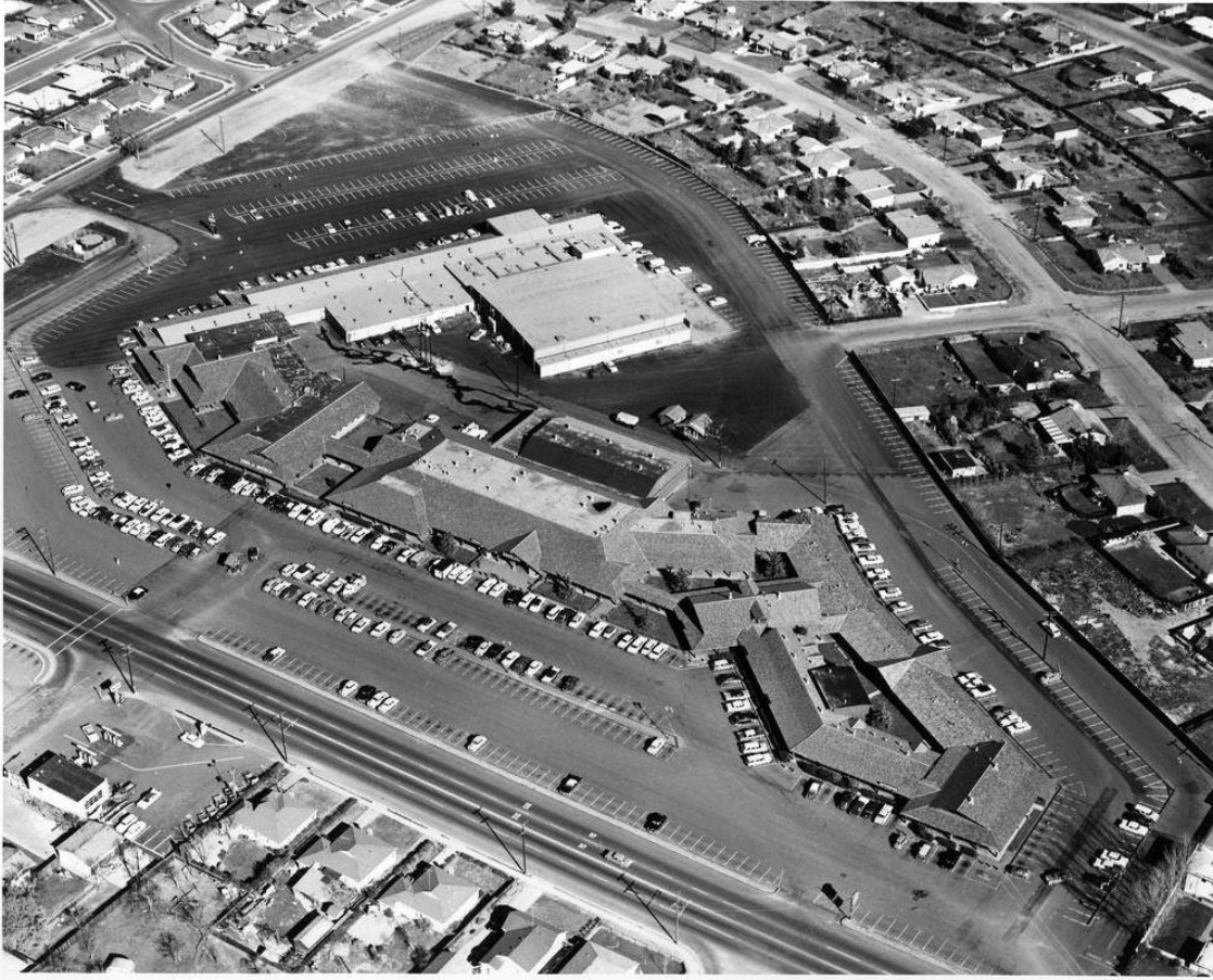
Aerial view (circa 1961) by Arnold Del Carlo. Photo reprinted with permission of Sourisseau Academy for State and Local History, San José State University. View from southwest.
