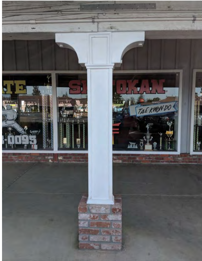
Typical Clad Column. July 2018.
