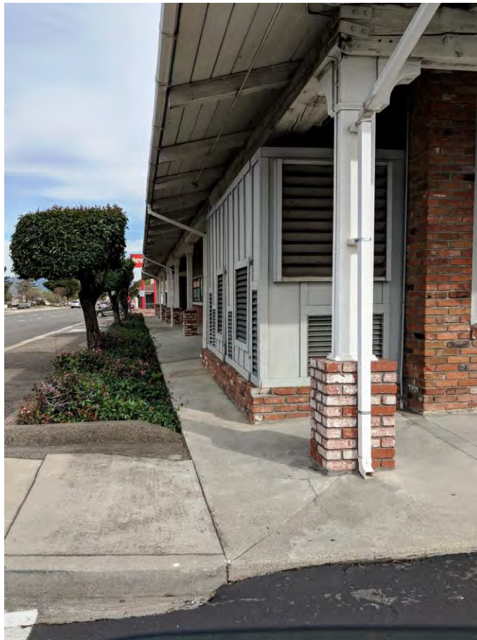
Typical Rear of Building Along Camden Avenue Sidewalk. Viewed facing East. July 2018.
