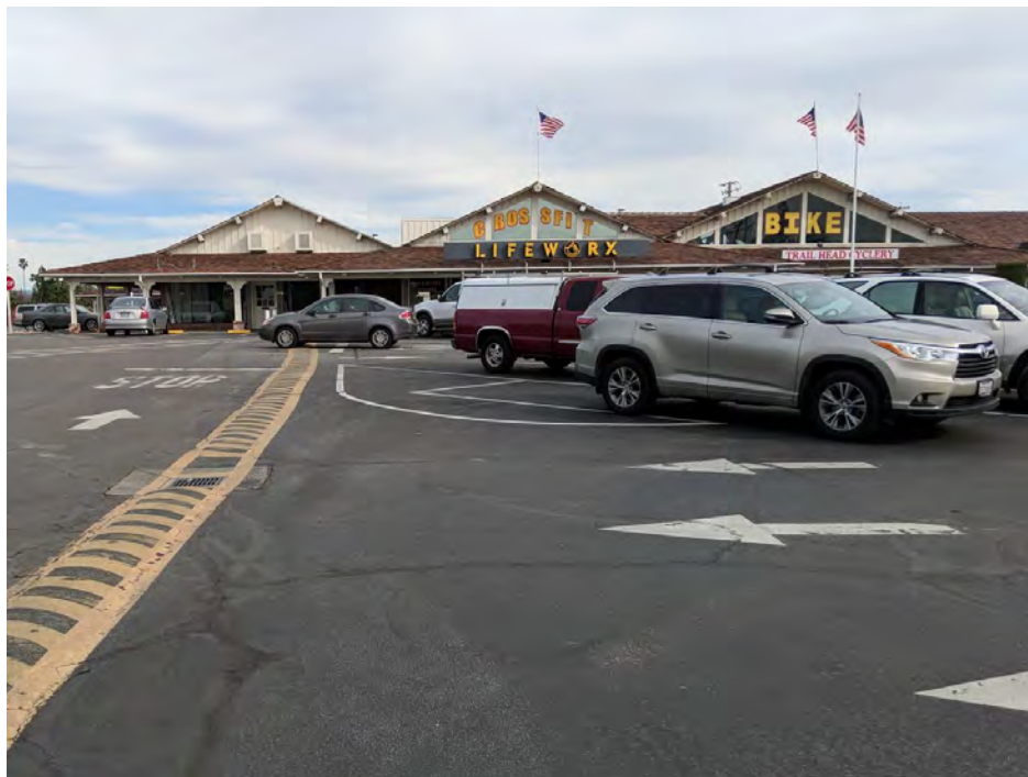
Northwest Corner of the Main Complex, With Three Gables. Viewed facing East. July 2018.
