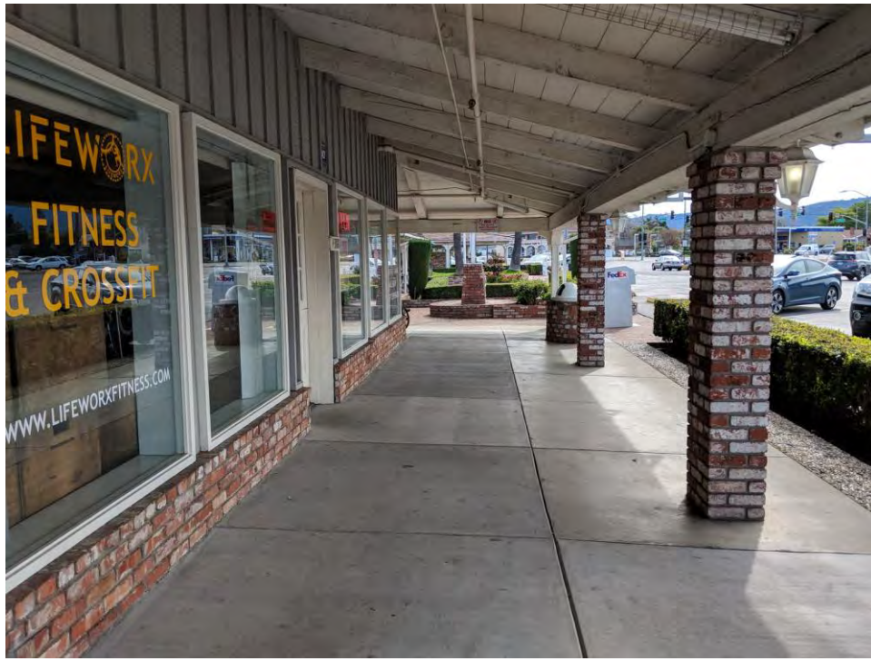
Corridor of North Wing, Facing Flagpole Feature. Viewed facing South. July 2018.
