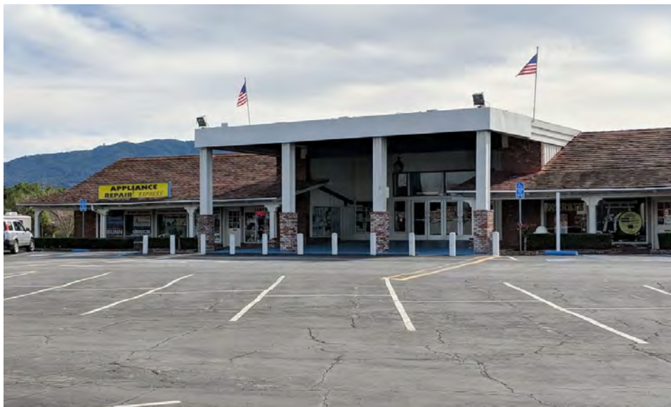
Bowling Alley Portico (Note altered fascia). Viewed facing Southeast. July 2018.
