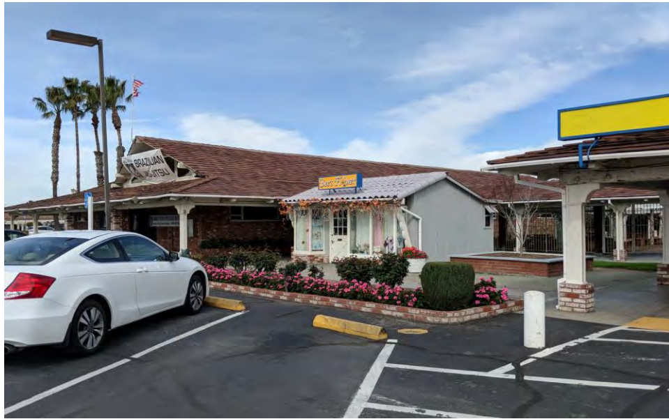
Courtyard Between Central Anchor Wing and North (Bowling) Wing, Featuring Detached Retail Shop. Viewed facing Northeast. July 2018.
