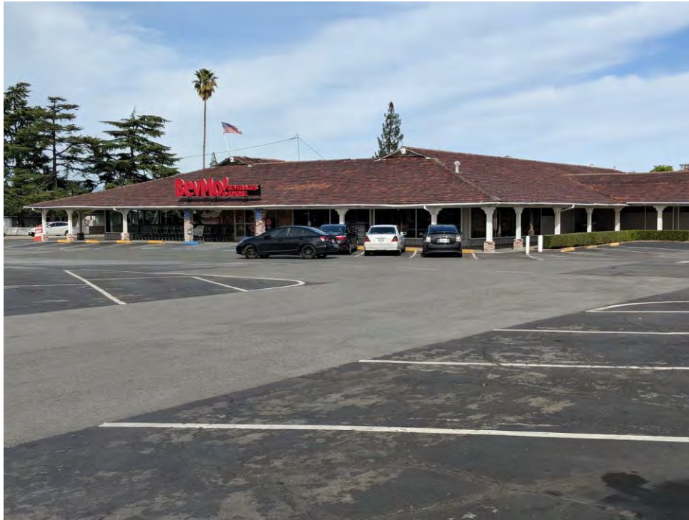
Northeast Corner Detached Retail Building, Anchor Space. Viewed facing Northeast. July 2018.
