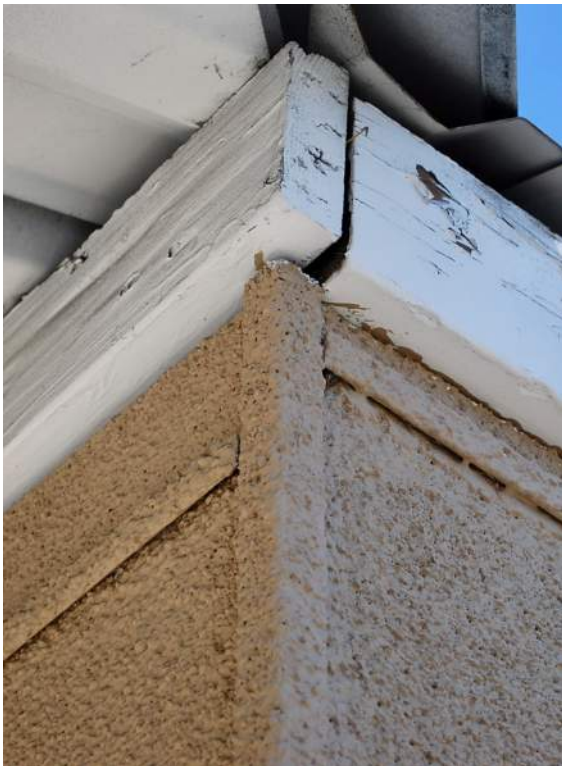
Here and on the following page are details of the plywood walls showing their construction. In some places they are held in place by metal strips, and in others by screws.
