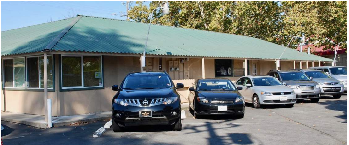
The rear (east) wall of the building
