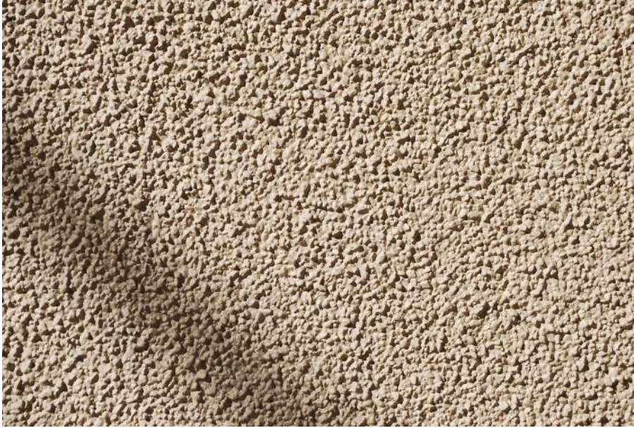
Detail of a plywood wall showing the surface texture.
