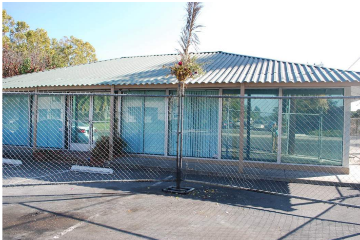
The south wing, 206 N. Bascom Avenue, with details below of the paired aluminum doors, aluminum windows, and sidelights.
