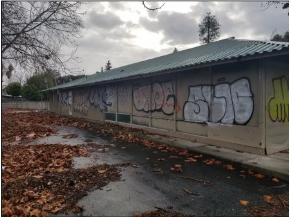
3 : View of the north side of the building.
