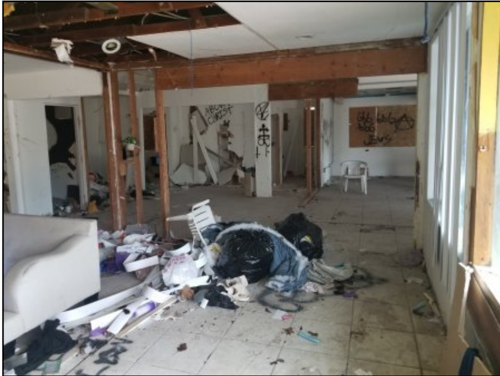
6 : View of the south interior of the building.
