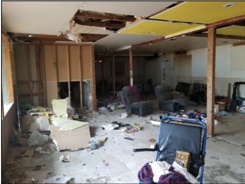
7 : View of the central interior of the building.
