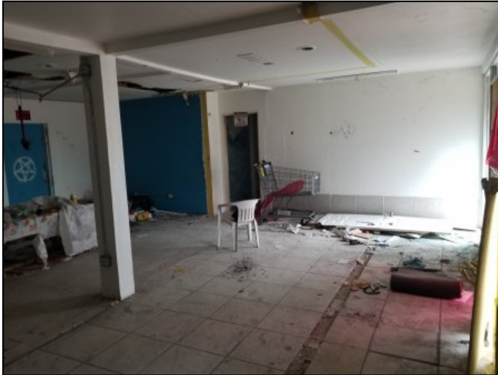
8 : View of the south interior of the building.
