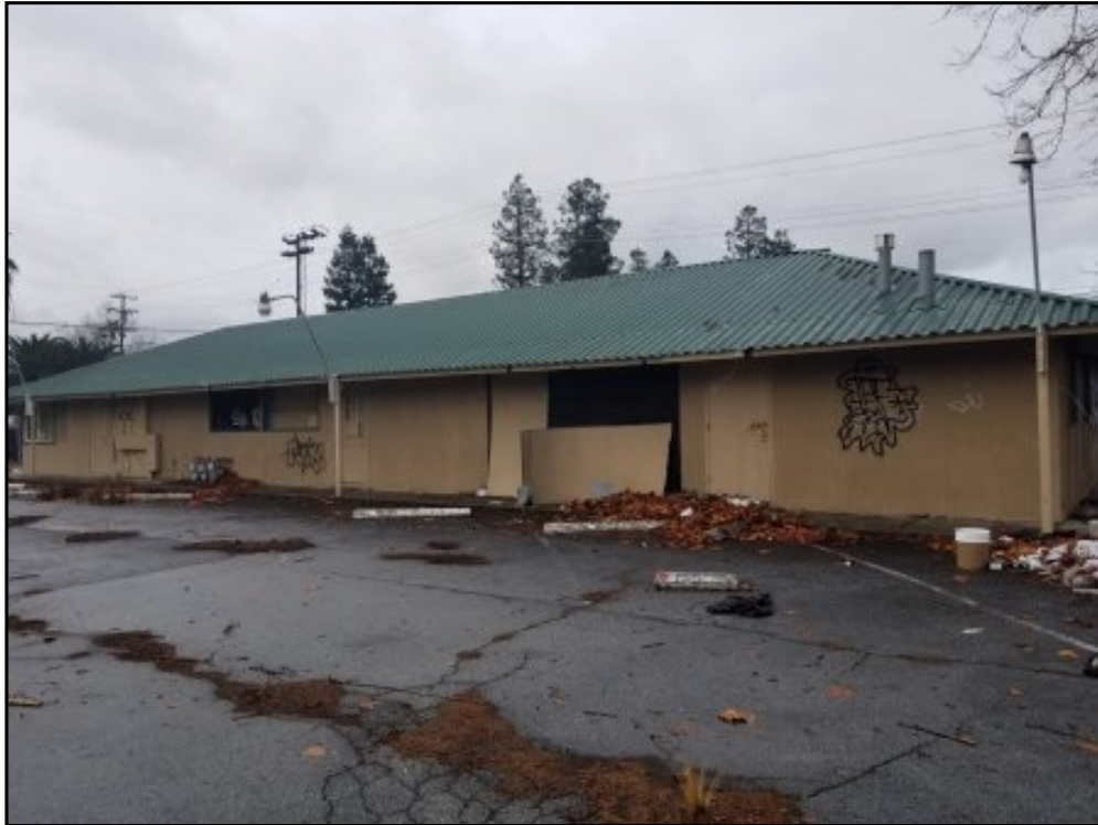
4 : View of the east side of the building.
