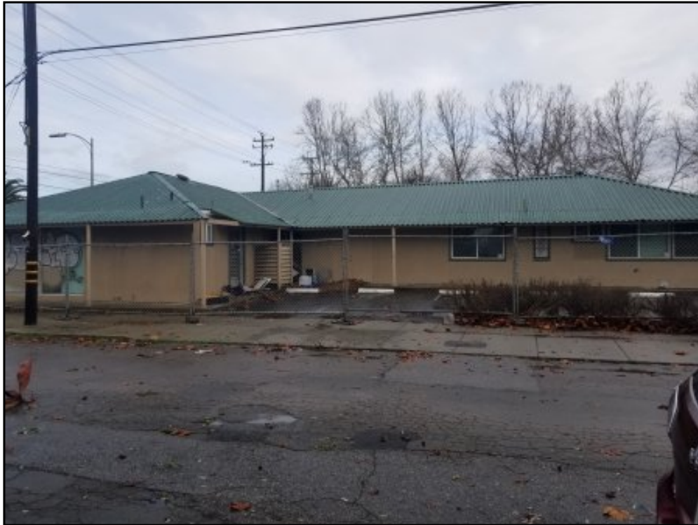
1 : View of the south side of the building.
