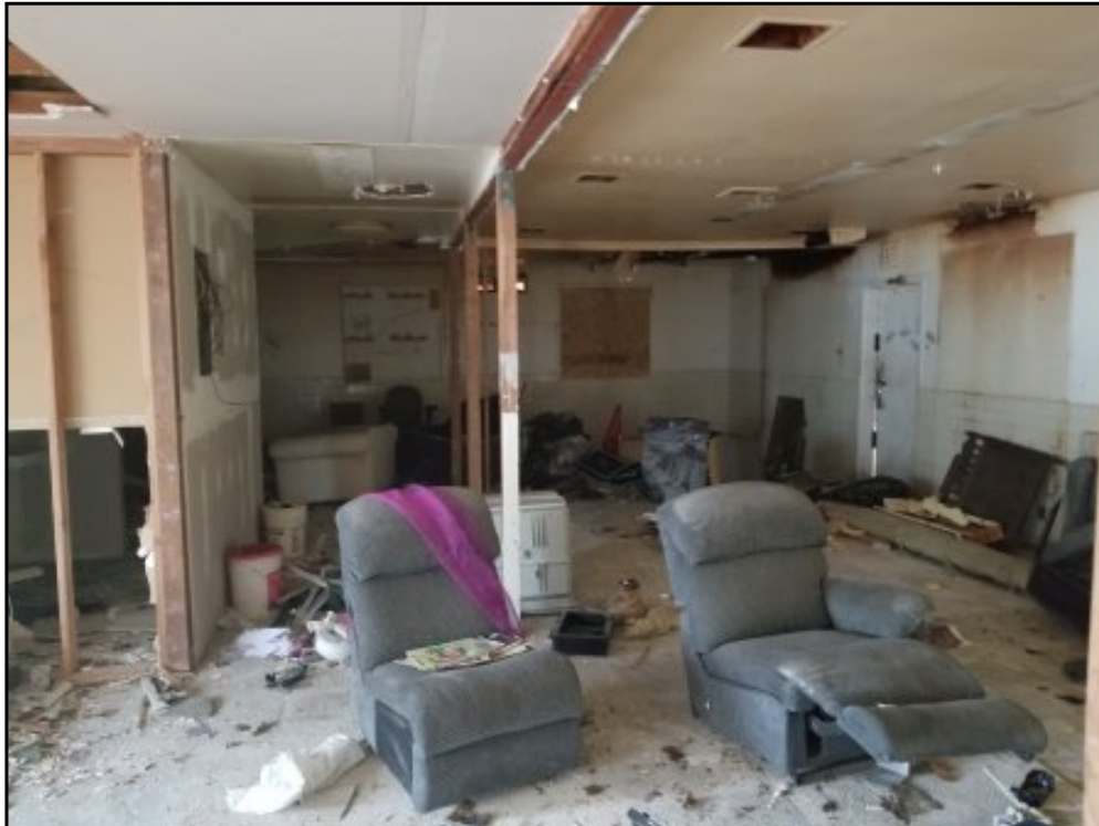
9 : View of the north interior of the building.
