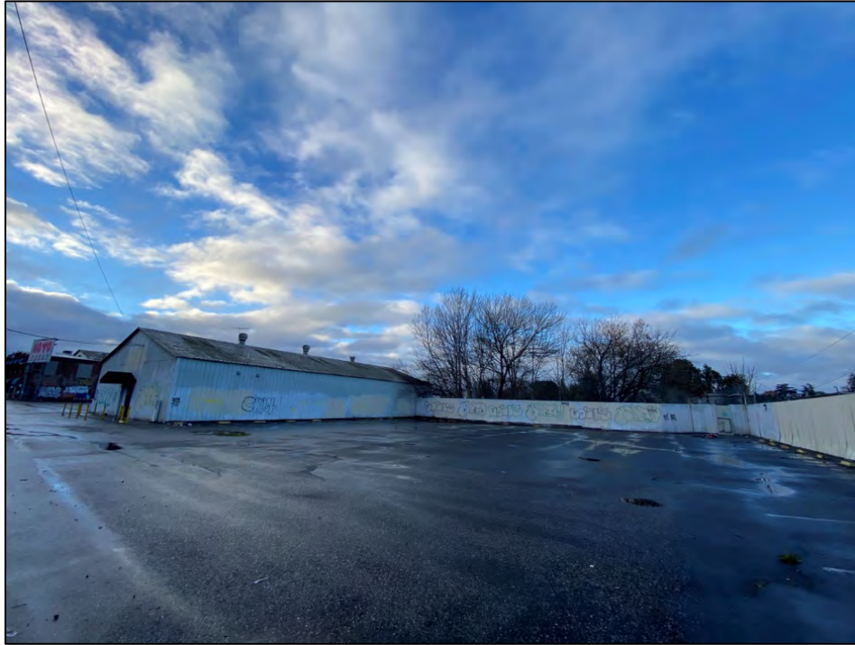
Photograph 9. Facing south in the northeast corner of the Project Site.
