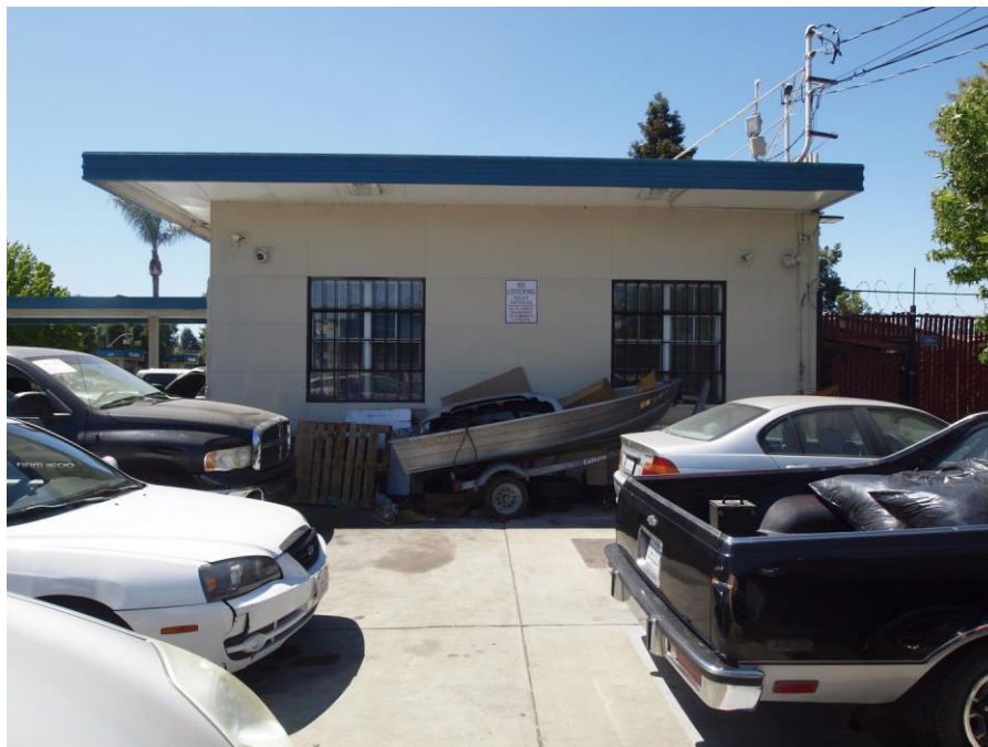
Side elevation of service bay area, viewed facing south
