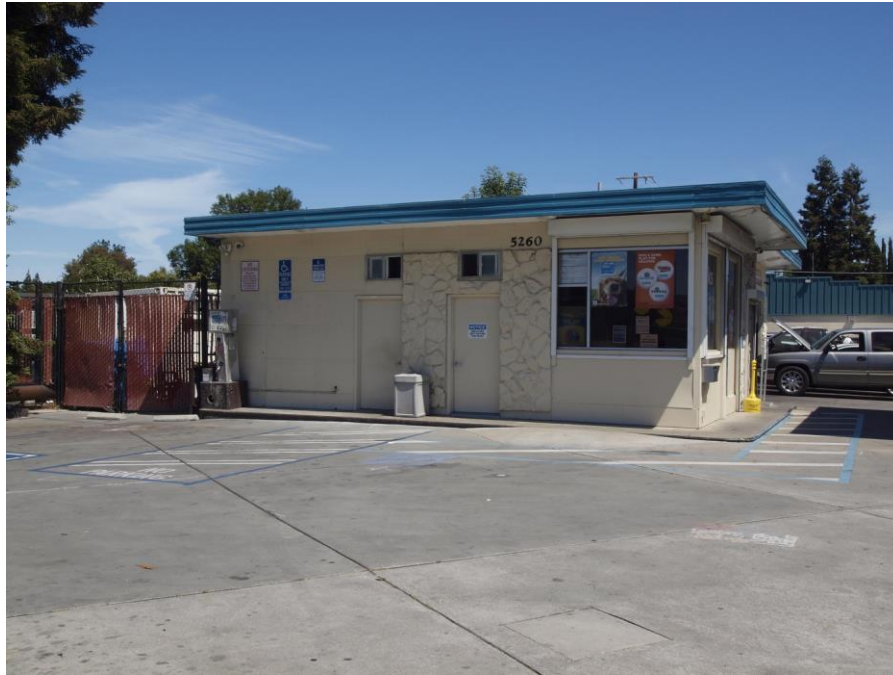
South elevation with stone veneer, viewed from Monterey Road facing north
