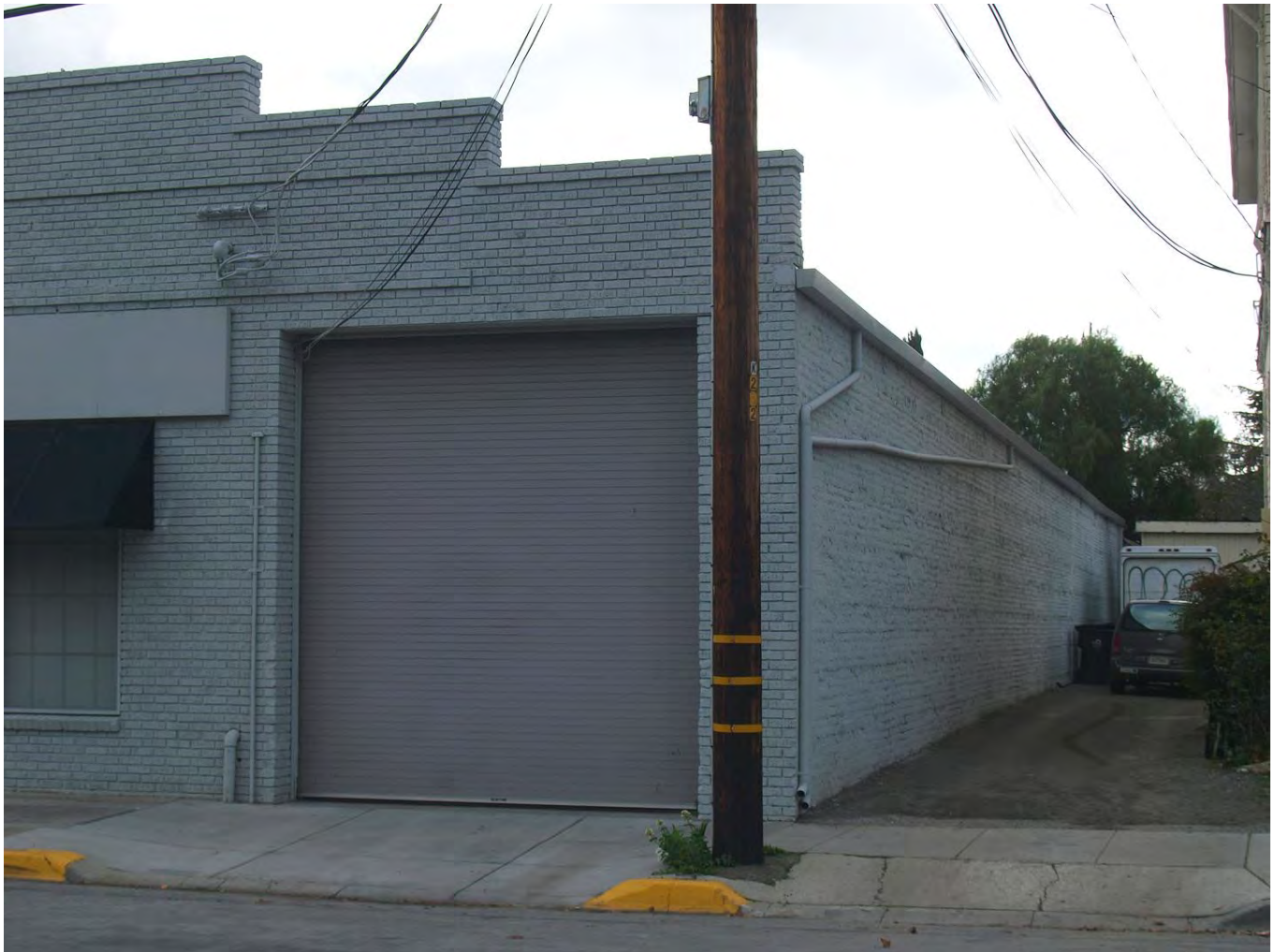
Detail view of garage door and north elevation at 151 North Autumn St., viewed facing southwest.
