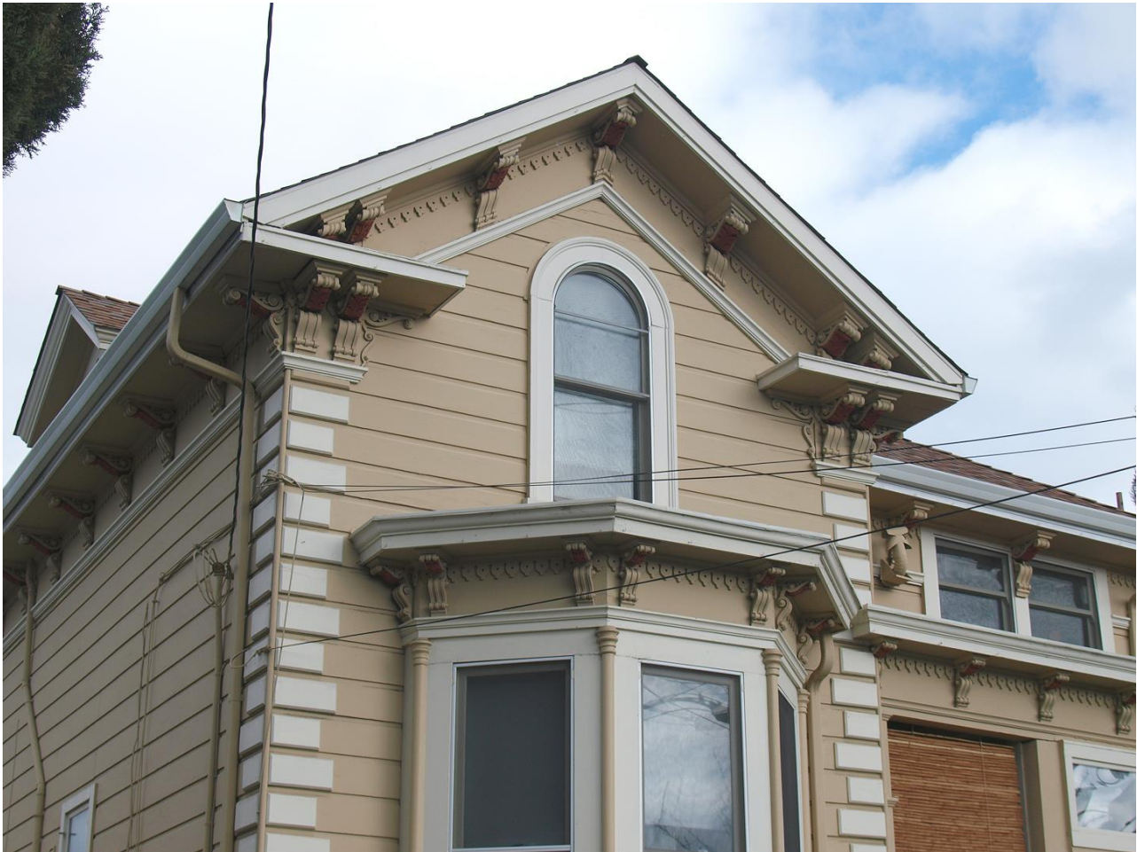
View of architectural detailing of 160 North Montgomery St., viewed facing east.
