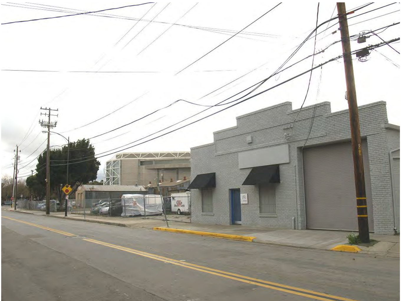
View of 151 North Autumn St. viewed facing south towards West St. John Street.
