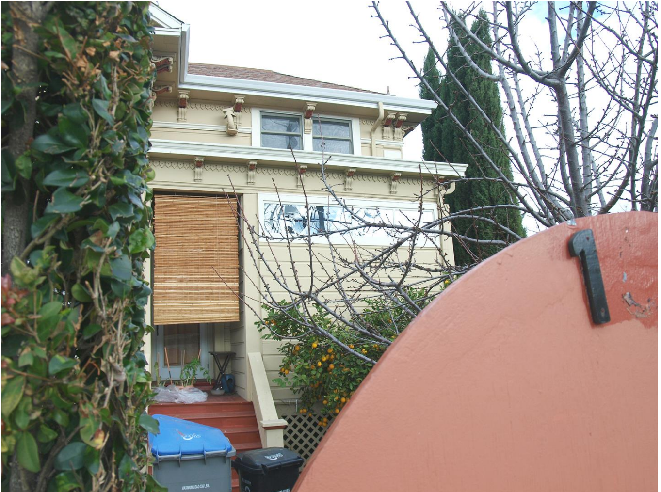
View of front porch of 160 North Montgomery St., viewed facing east.
