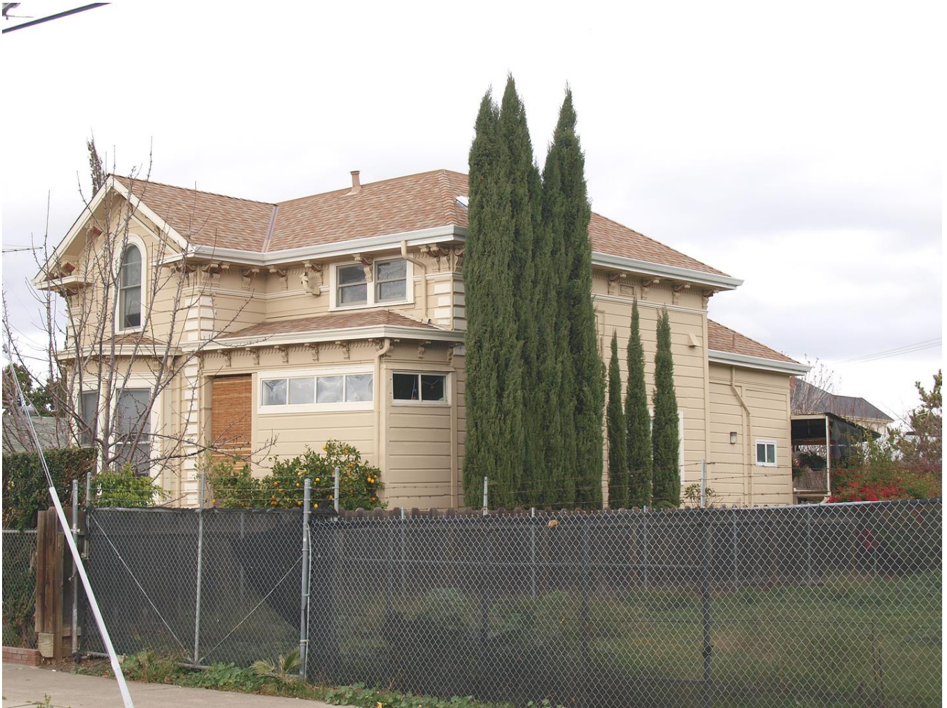
Side view of 160 North Montgomery St. including the adjacent vacant lot at 150 North Montgomery St., viewed facing northeast.
