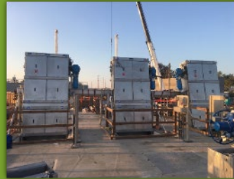
Three climbing bar screens installed at the Headworks Project.
