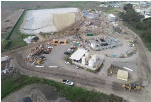
November 2021 aerial view of the Headworks Project.
