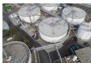
Completed paving at the Digester and Thickener Facilities.
