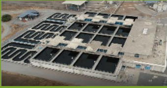
Aerial view of the current filtration area.
