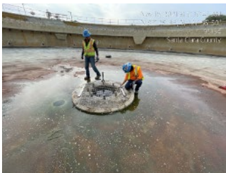
Contractor installing a screen in a clarifier
