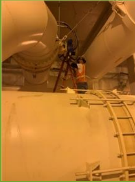
Contractor installing a new electric actuator in the PEPS Building.
