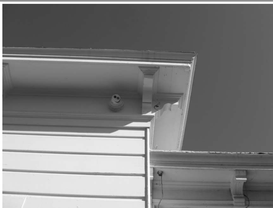
Photo 8: Detail of boxed and enclosed eaves with decorative brackets.
