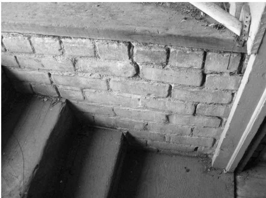
Photo 34: Detail of brick foundation in basement entry.
