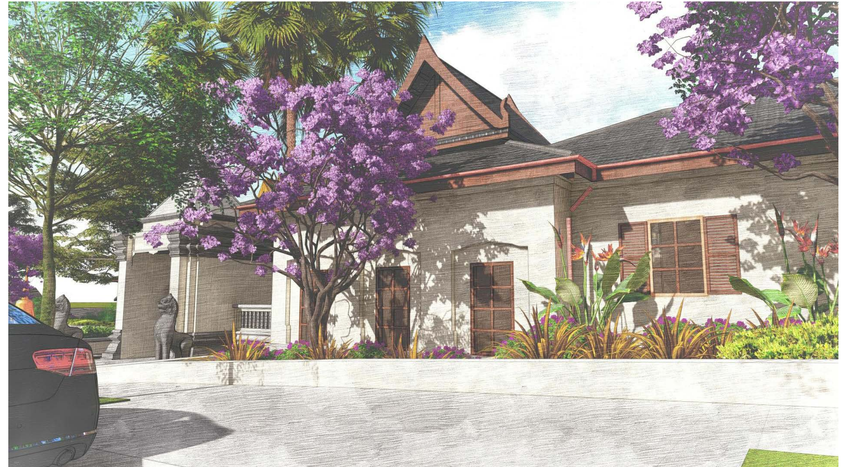
VIEW OF ENTRY GATE & CLASSROOM AT EYE LEVEL FROM NORWOOD AVENUE (RENDERED VIEW ALSO LOCATED ON SHEET G7.2)
