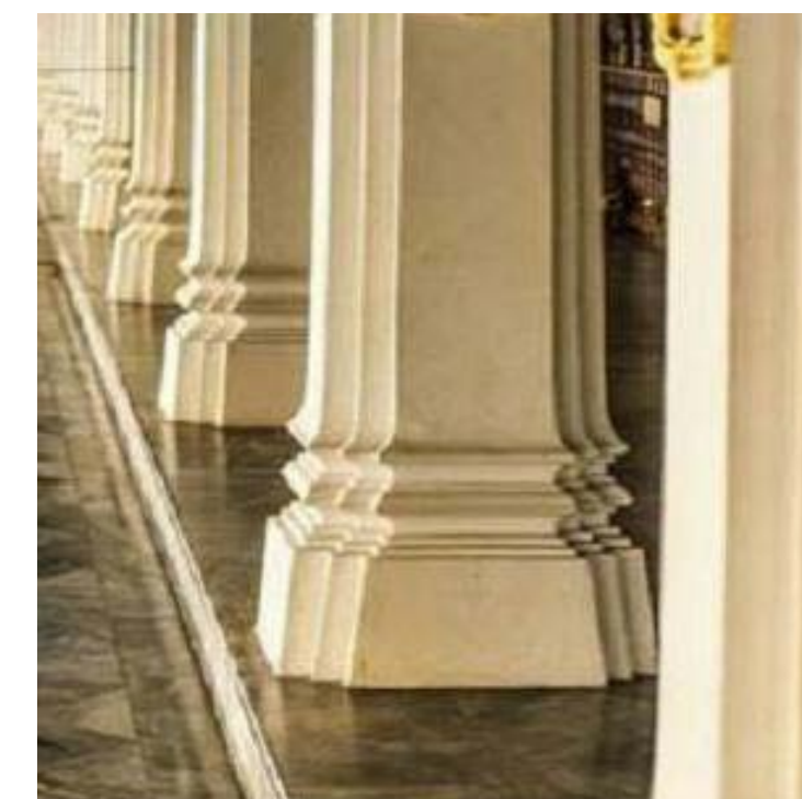
16 PAINTED PLASTER COLUMN WITH STONE BASE
