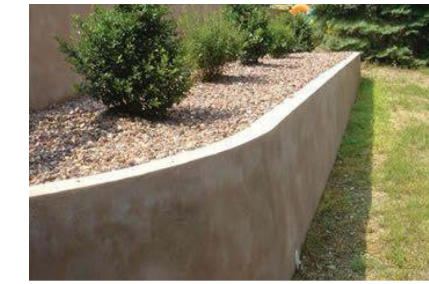
L12 PAINTED PLASTER RETAINING WALL
