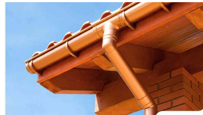
08 PAINTED WOOD FASCIA & EAVE, COPPER GUTTERS
