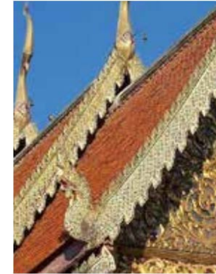
11 DECORATIVE WOOD BARGE BOARD AT ROOF TIERS, ADORNED WITH FINIALS, PAINTED & GILDED
