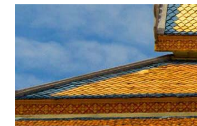
25 DECORATIVELY PAINTED FASCIA AND EAVE
