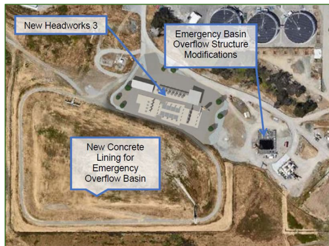
FIGURE 18 SITE FOR NEW HEADWORKS
