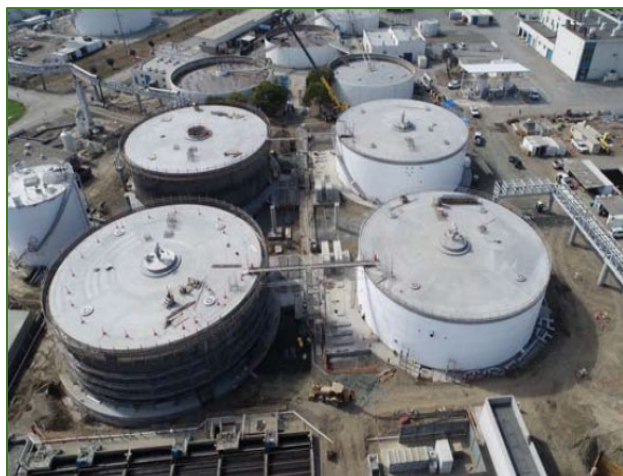
FIGURE 25 AERIAL IMAGE OF PROGRESS ON UPGRADES TO DIGESTERS 5 - 8
