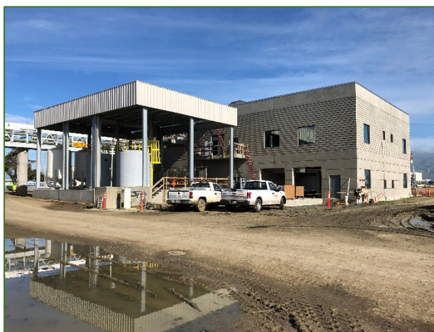
FIGURE 24 NEW SLUDGE SCREENING BUILDING WAS COMPLETED IN 2021
