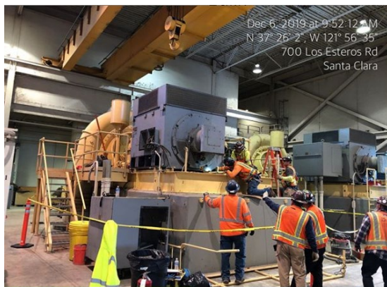
FIGURE 16 BLOWER IMPROVEMENTS PROJECT PREPARING TO INSTALL A NEW ELECTRIC MOTOR TO IMPROVE THE AERATION SYSTEMS’ RELIABILITY
