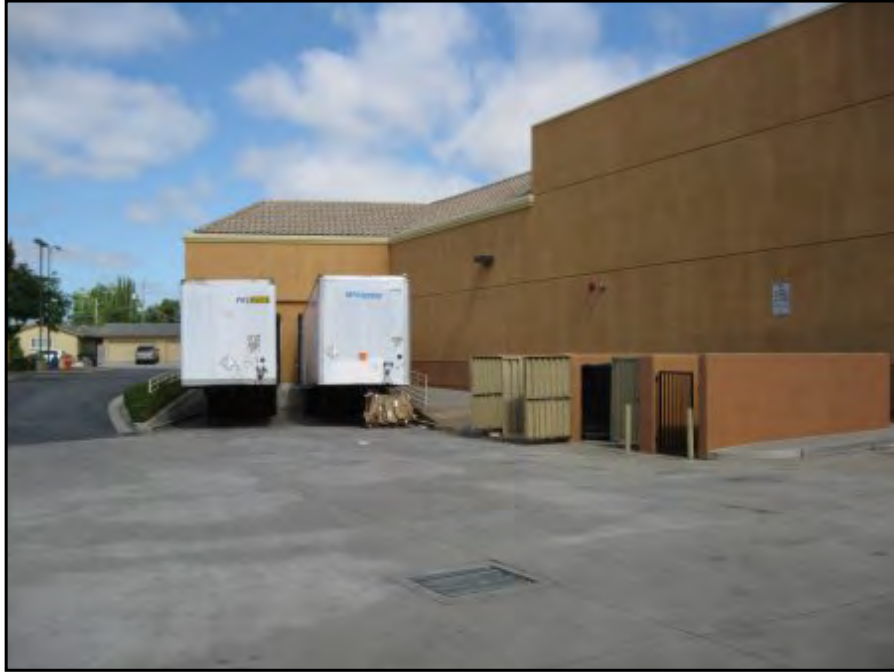
Loading dock at rear of Dick's Sporting Goods.
