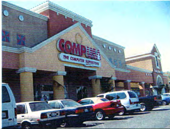
Photo #7: Front view of multi-tenant structure
