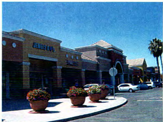
Photo #6: Front view of multi-tenant structure
