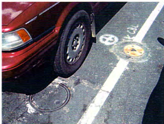
Photo #21: Typical groundwater monitoring wells observed at Union 76 gas station
