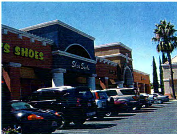
Photo #5: Front view of multi-tenant structure
