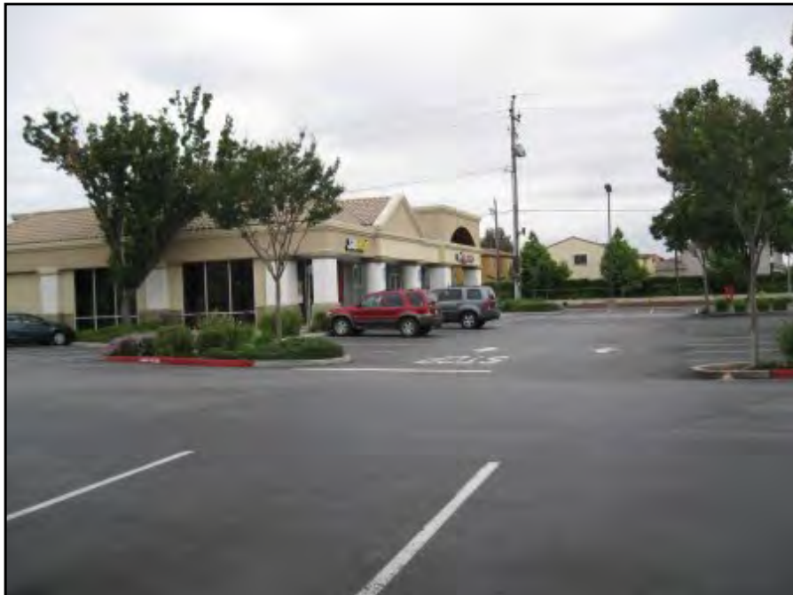
Subway and Verizon (684/686)
