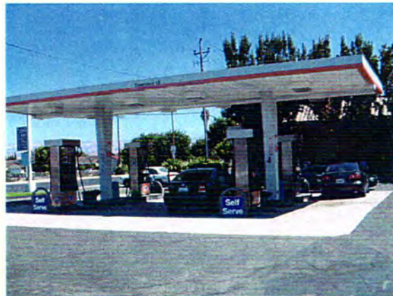
Photo #17: Fuel dispensers at Union 76 gas station
