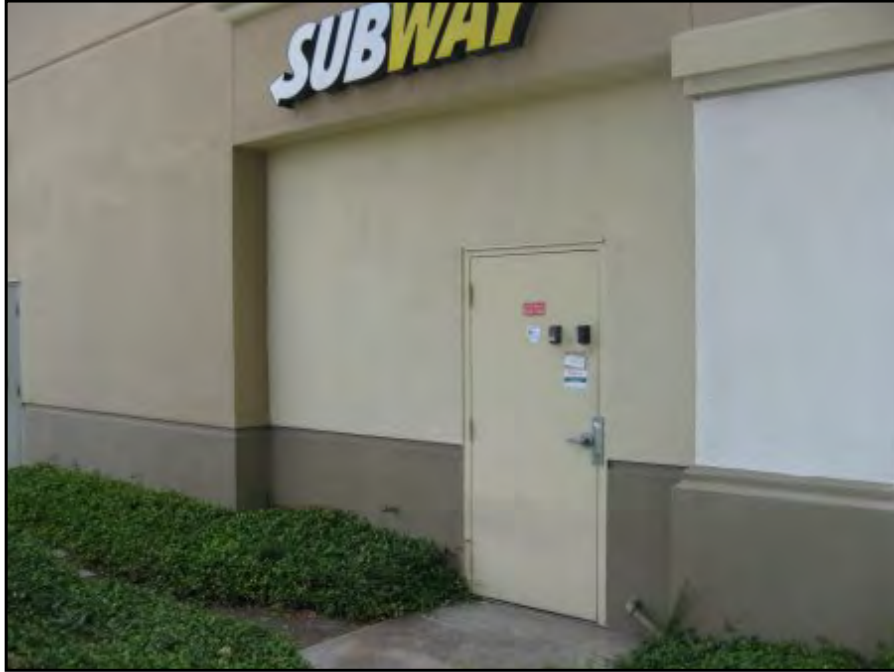
Interior rear of Subway (684)
