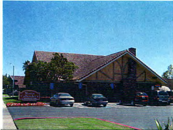
Photo #2: Exterior view of Marie Calendar's structure
