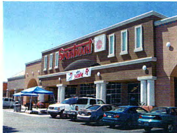
Photo #10: Exterior view of Sportmart structure
