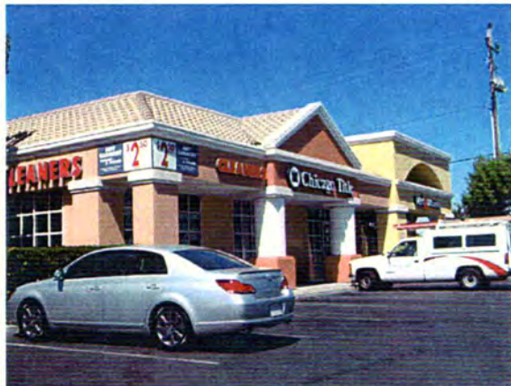
Photo #9: Front view of multi-tenant structure
