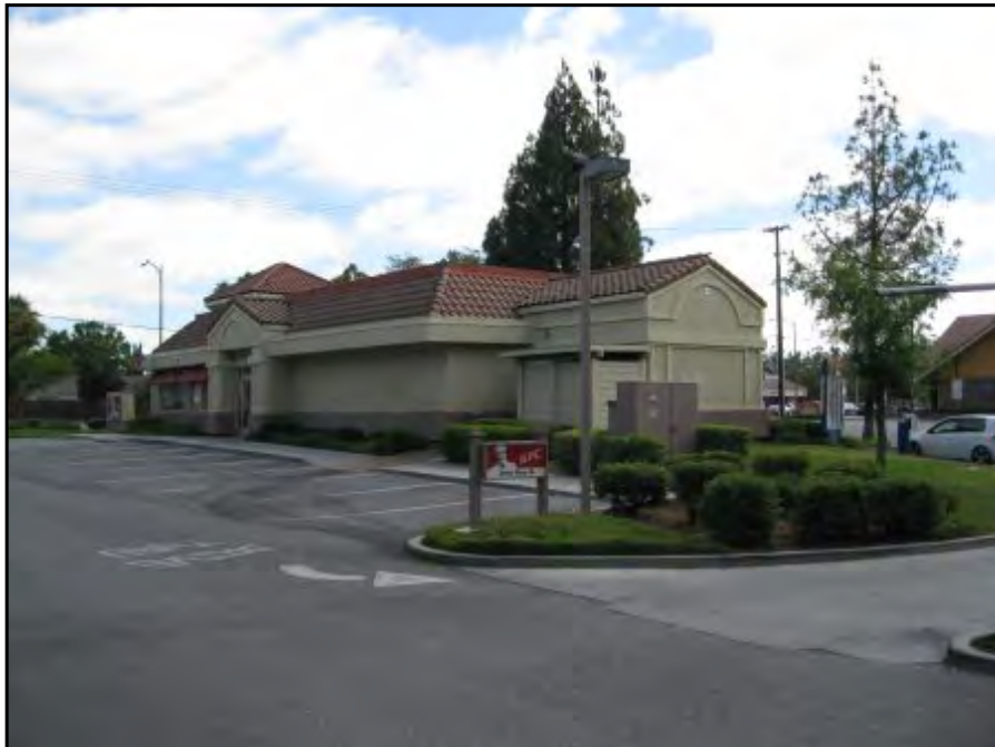
Exterior of KFC showing pad-mounted transformer.
