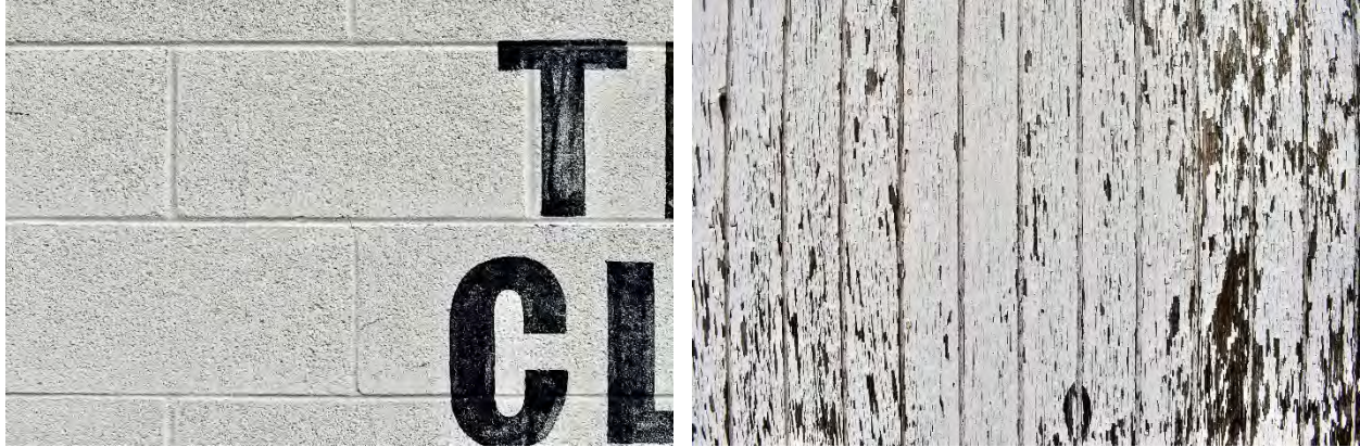
Exposed concrete blocks (left), T-111 vertical wood siding (right)
