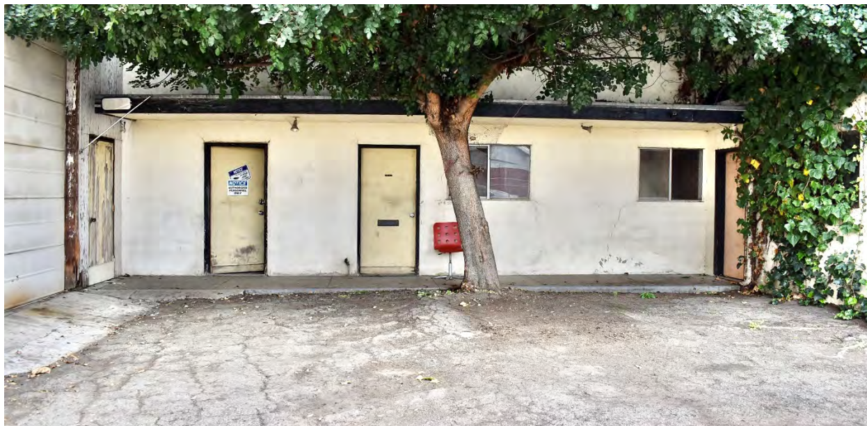
Figure 16: Office wing exterior
