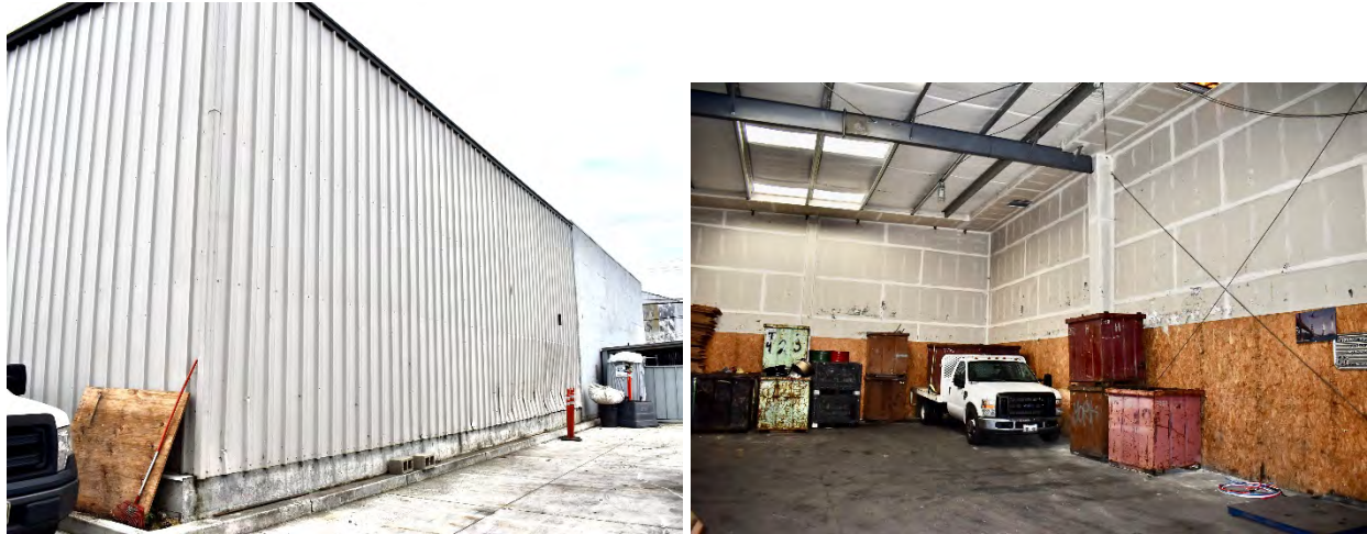
Figure 22: north side, perspective view toward front (left), rear addition from 2008 (right)
