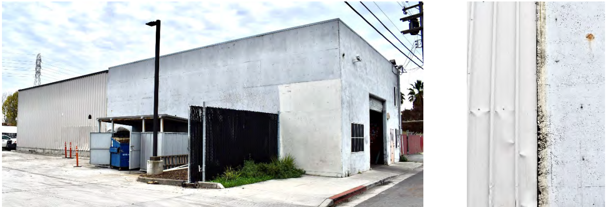
Figure 19: 254 McEvoy showing back metal and front concrete halves (left); close-up of materials (right)
