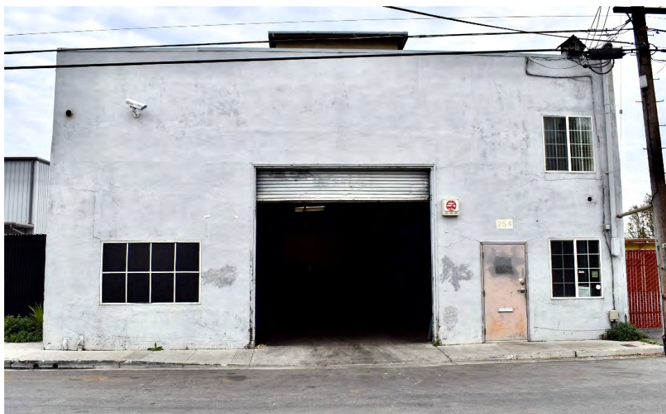
Figure 20: Street View of 254 McEvoy showing doors and windows
