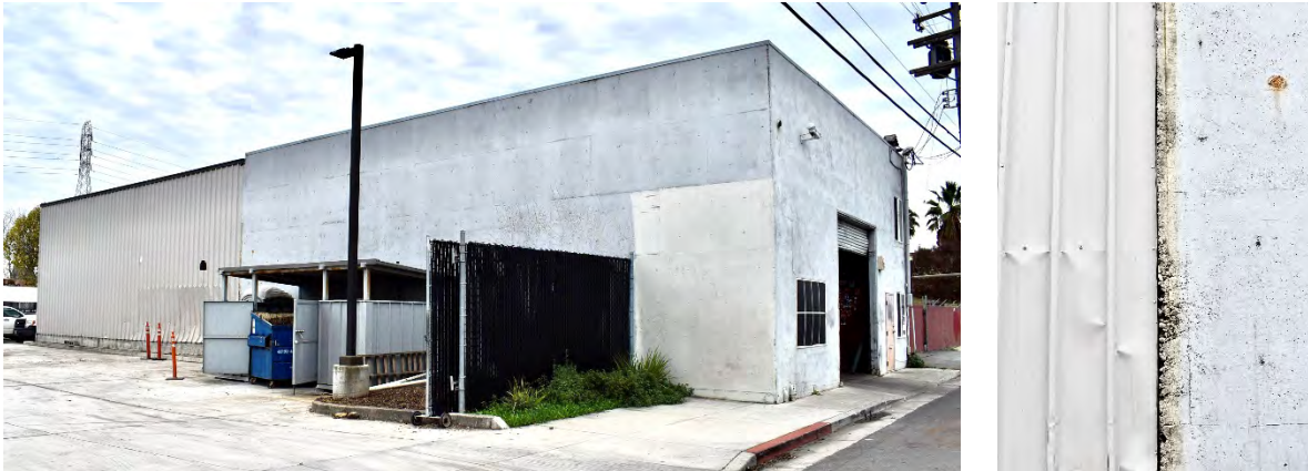
254 McEvoy back metal and front concrete (left); close-up of materials (right)
