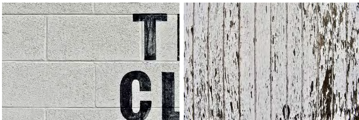
Figure 12: (left) exposed concrete blocks, (right) T-111 vertical wood siding
