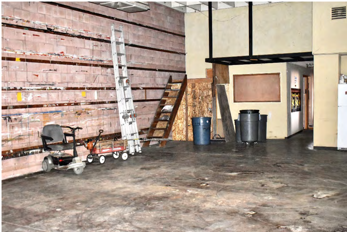
Warehouse looking south toward the offices
