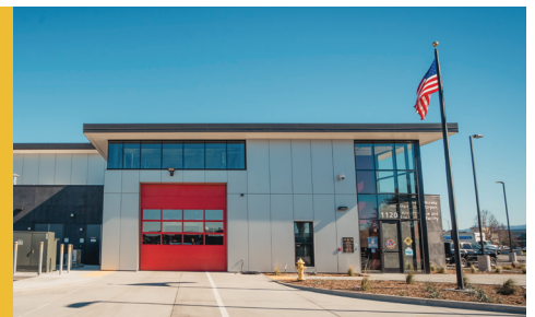
Exterior view of public-facing apparatus bay.
