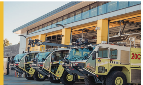
Exterior view of airport-facing apparatus bay.
