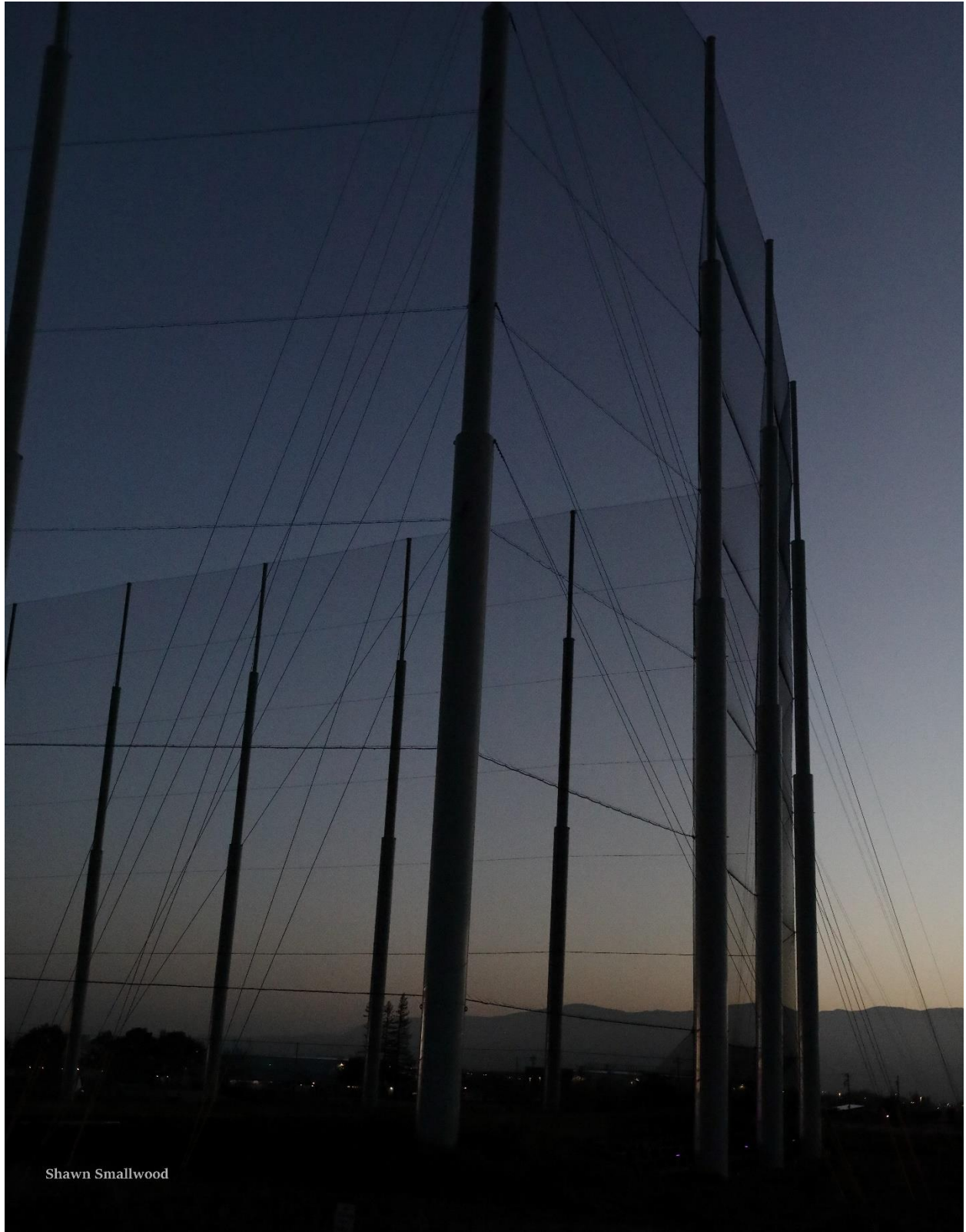
Photo 29. The TopGolf net viewed towards the glow of the rising sun at 06:42 hours, 1 April 2022. Note that the net would be less visible when viewed from the north or east. Also note that the guy cables are unmarked, and no markers are on the net.
