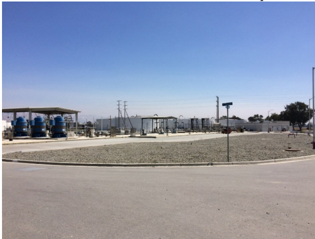
Proposed Site for New Headworks
