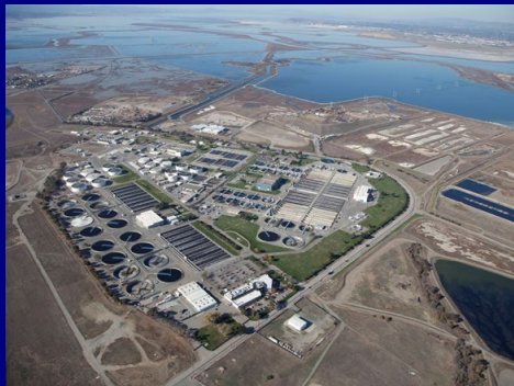
Water Pollution Control Plant
