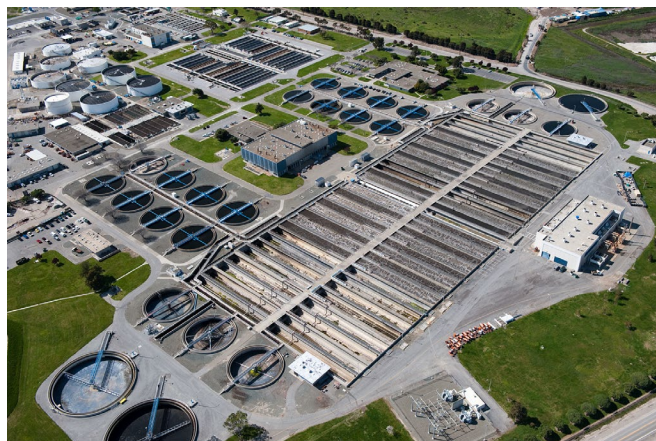
San José-Santa Clara Regional Wastewater Facility
