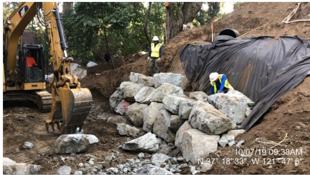
An outfall being rehabilitated on Thompson Creek
