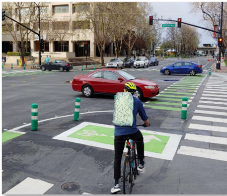
Quick Build Safety Improvements at W San Fernando St and Almaden Blvd
