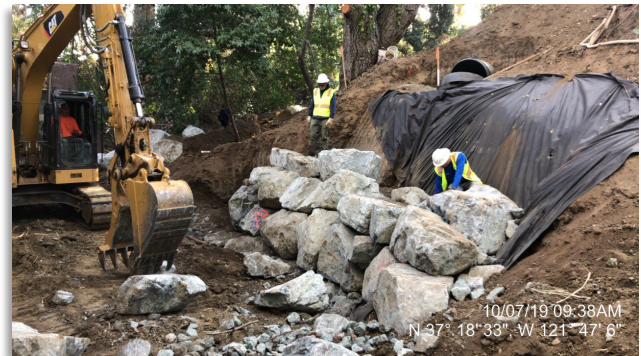
An outfall being rehabilitated on Thompson Creek
