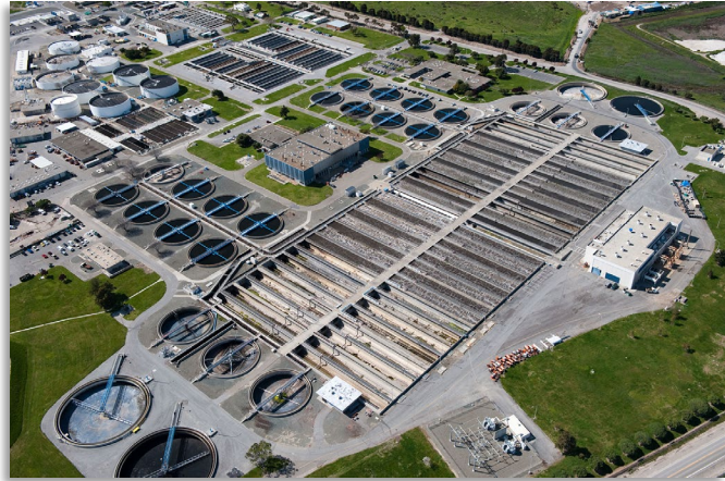
San José-Santa Clara Regional Wastewater Facility
