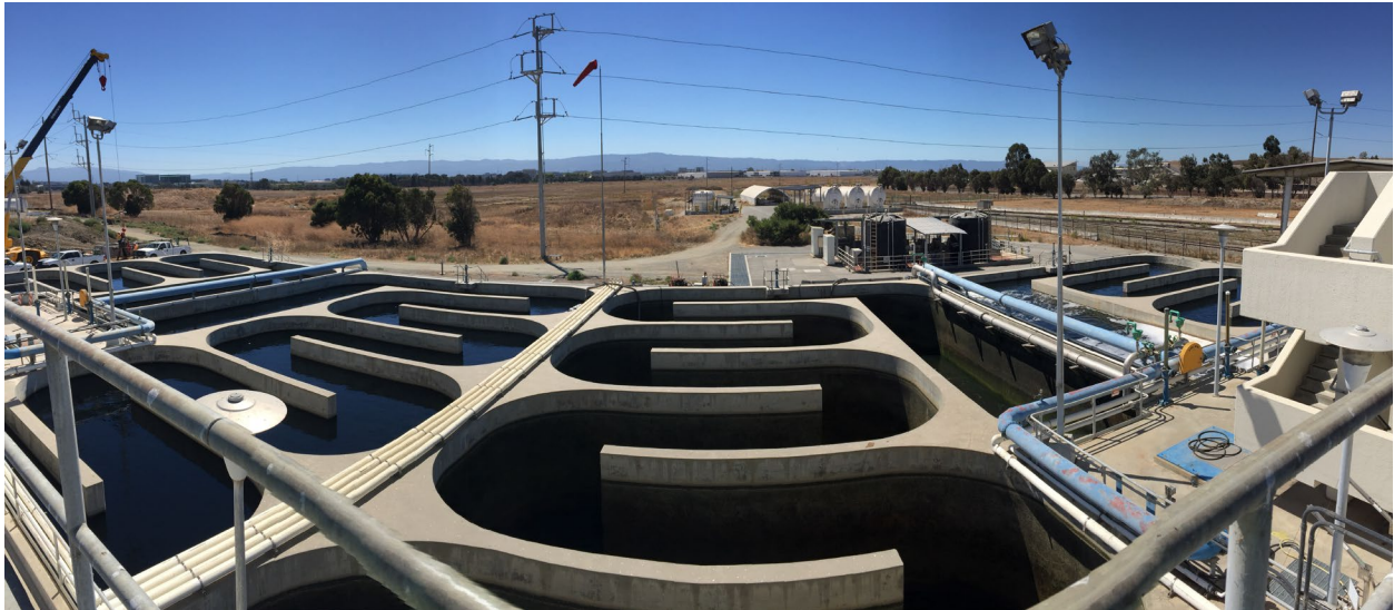
Existing Filtration Structure
