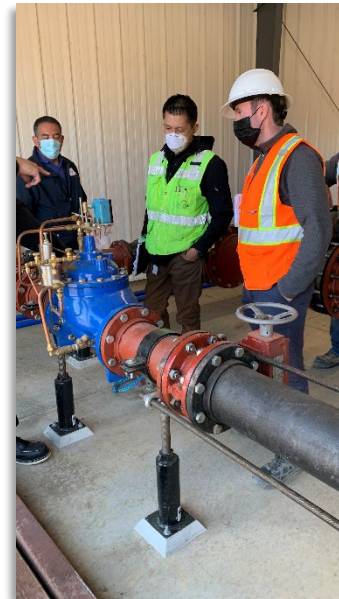
City staff and contractor discuss a newly installed control valve
