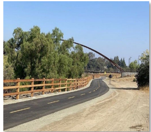
Coyote Creek Trail (near HHPZ Bent Bridge)
