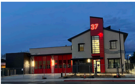
Completion of Fire Station 37
