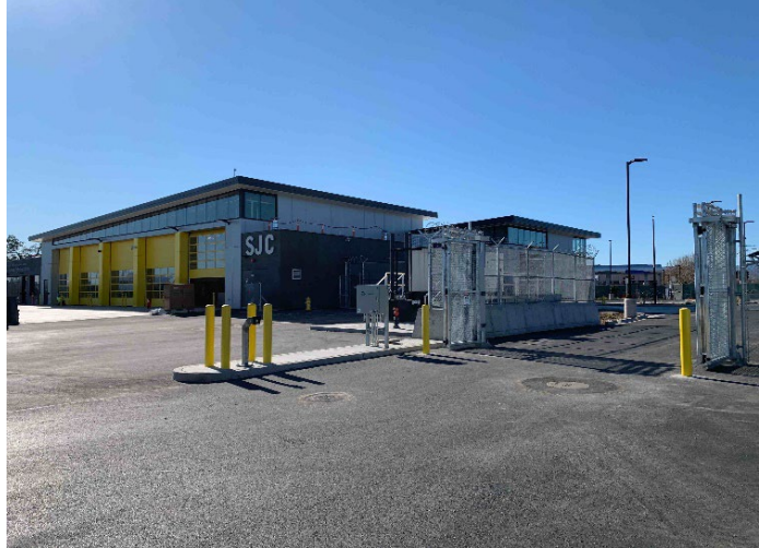
Aircraft Rescue and Fire Fighting Facility
