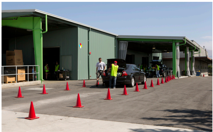
Another view of the facility at 1608 Las Plumas, San Jose. (LiPo Ching/Bay Area News Group)
