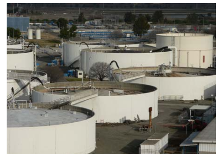
Water Pollution Control Plant – Digester Tanks
