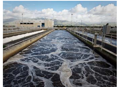
Aeration Basin for the Activated Sludge Process
