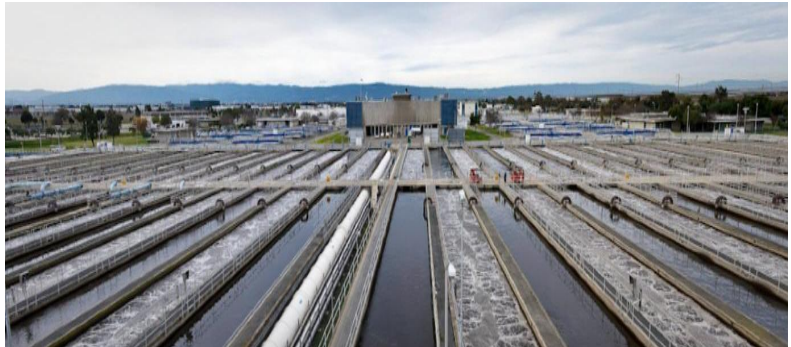
Aeration Basin for the Activated Sludge Process Photo by Robert Dawson
