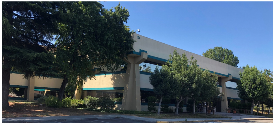
The north façade.
