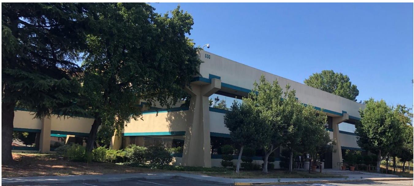
Figure 2. The north façade.
