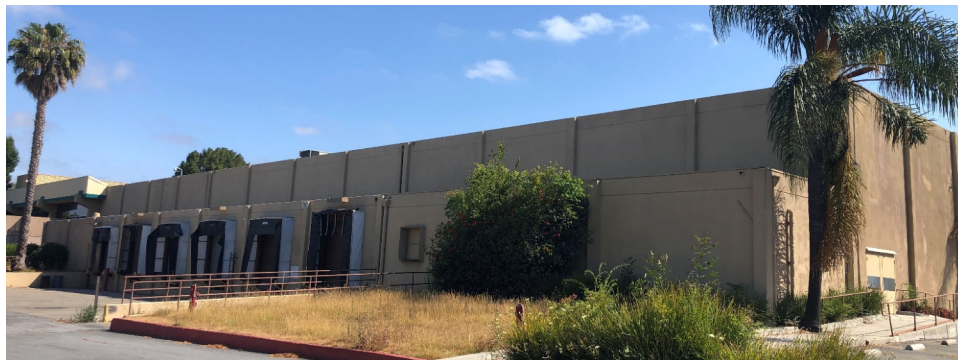
The partial west façade.
