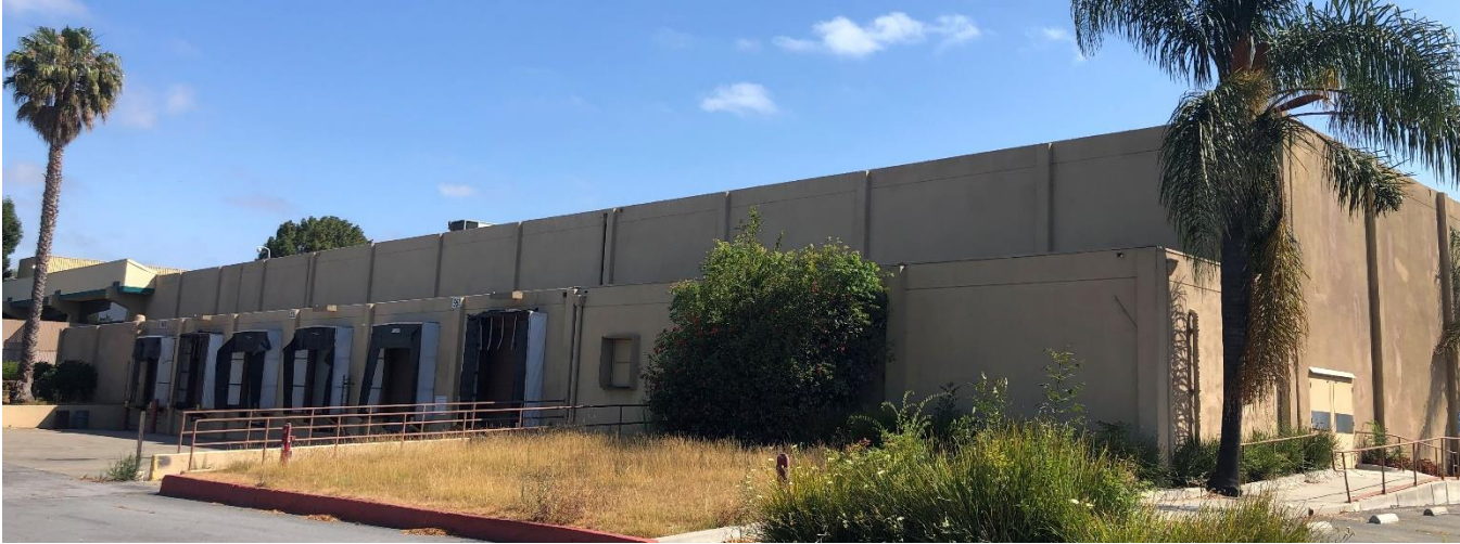
Figure 3. The partial west façade.
