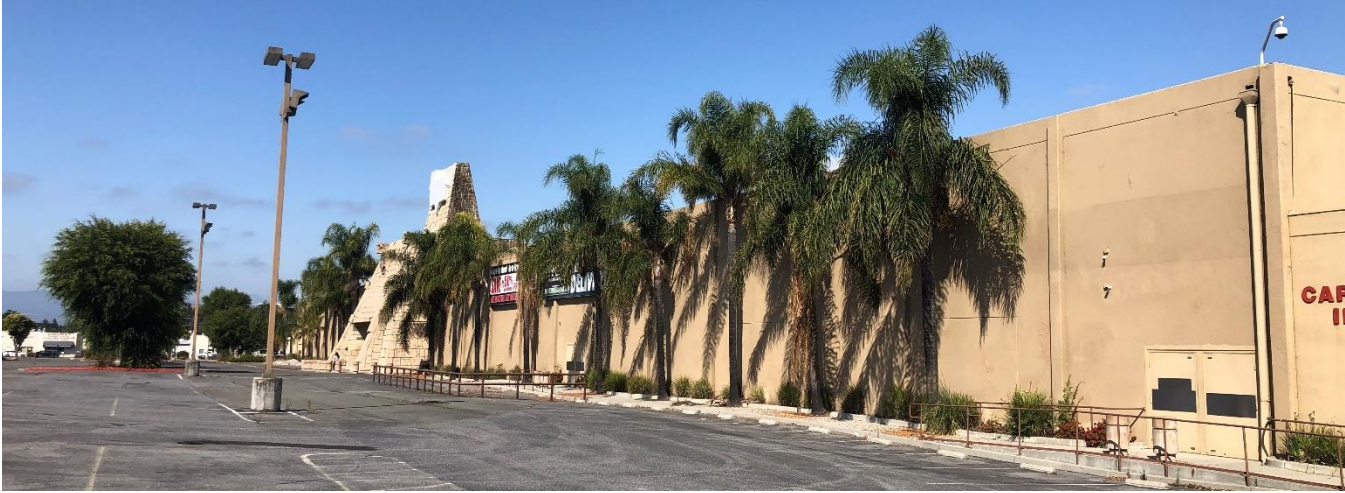
Figure 4. The south façade.
