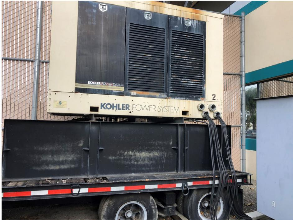
**Photograph 11:** Emergency generator with self-contained 250-, 750-, and 800-gallon diesel aboveground storage tanks on the western Site building exterior.
