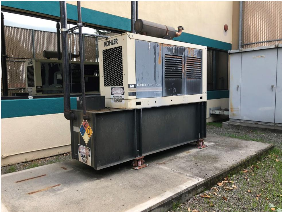
**Photograph 10:** Emergency generator with self-contained 250-, 750-, and 800-gallon diesel aboveground storage tanks on the western Site building exterior.
