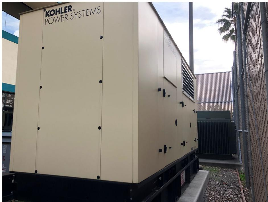
**Photograph 12:** Emergency generator with self-contained 250-, 750-, and 800-gallon diesel aboveground storage tanks on the western Site building exterior.
