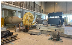
New motor installed on Secondary Blower #2
