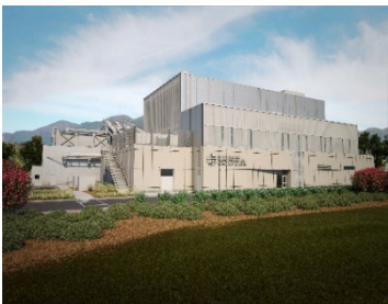
The new dewatering facility (rendering above) will use centrifuges to dry the digested sludge, and features a load-out facility to haul solids for additional processing and beneficial reuse application
