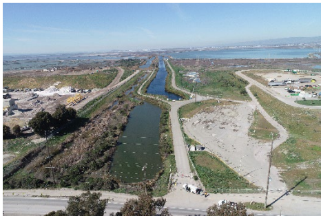
January 2022 aerial view of the Outfall Channel and Instrumentation Improvements Project.
