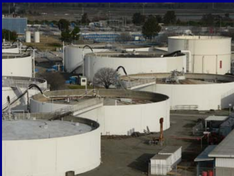
Digester Rehabilitation Project
